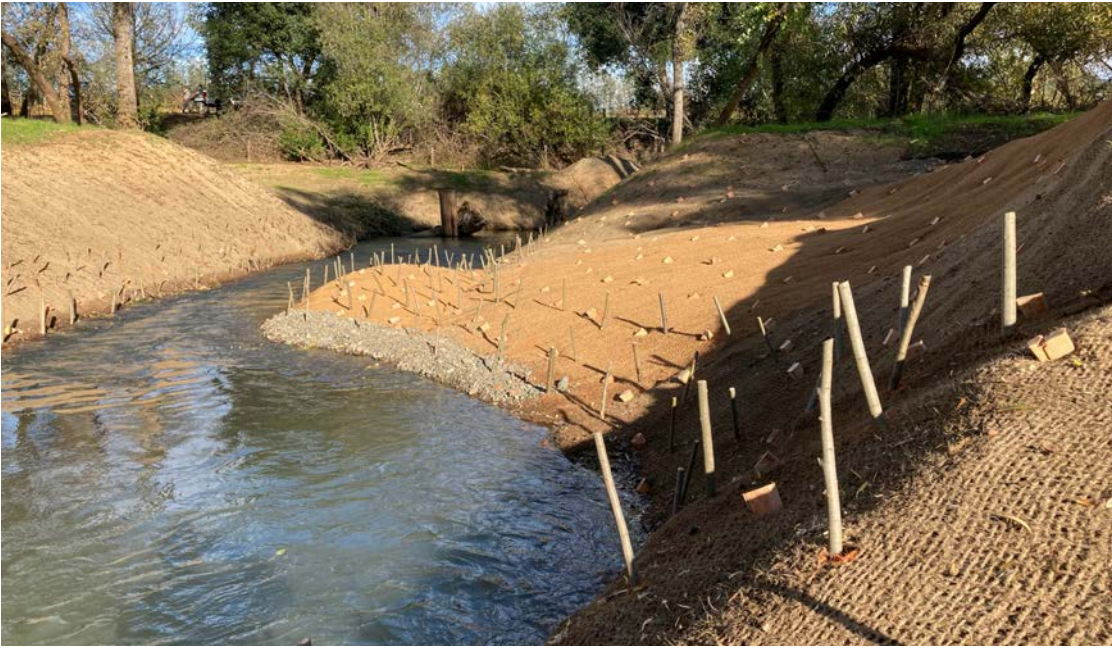
Repair of minor bank failure area showing new fabric, willow cuttings and wooden stakes at inlet to the Phase III Reach 5A site (repair area is on right hand side of photo). View is looking downstream into the habitat feature. Photo taken November 17, 2021.
