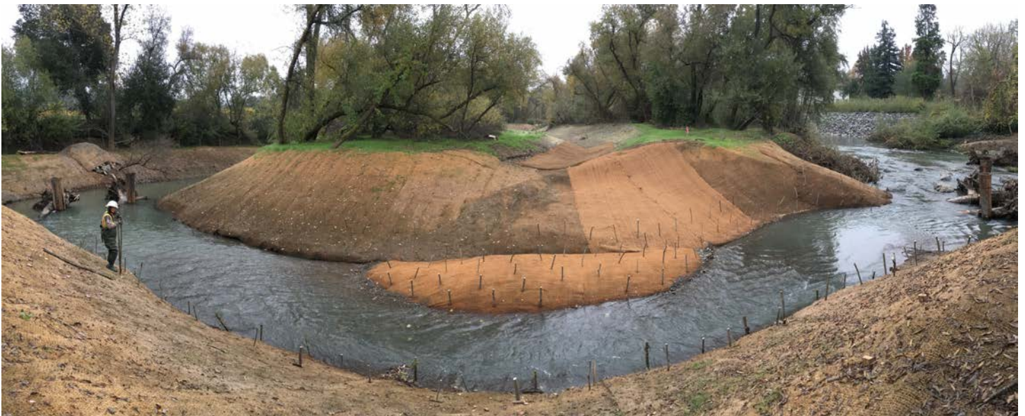
Another view of inlet channel on November 15 during the restaking of the fabric, showing the pool and riffle that were created by the bank adjustment and gravel deposition. The mainstem of Dry Creek is on the right and flow is going right to left into the habitat feature. Juvenile salmon were feeding at the downstream end of the inlet riffle by the log structures.
