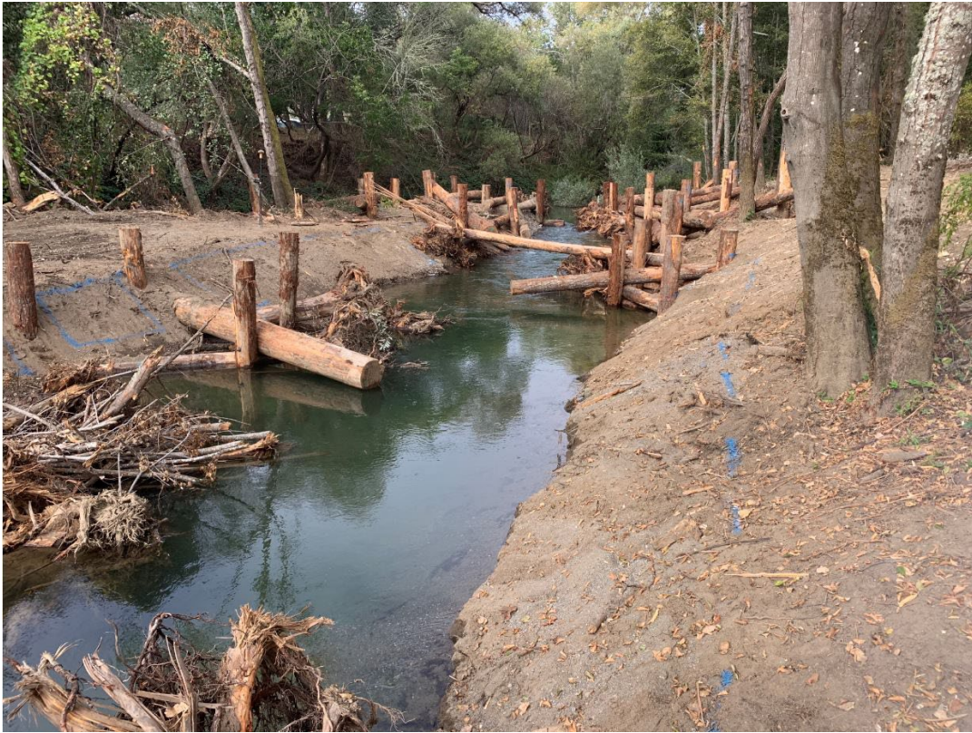
Looking upstream at the upstream end of the nearly completed Dry Creek Reach 13A Site. All that remains is installation of erosion prevention fabric in the areas outlined in blue.
