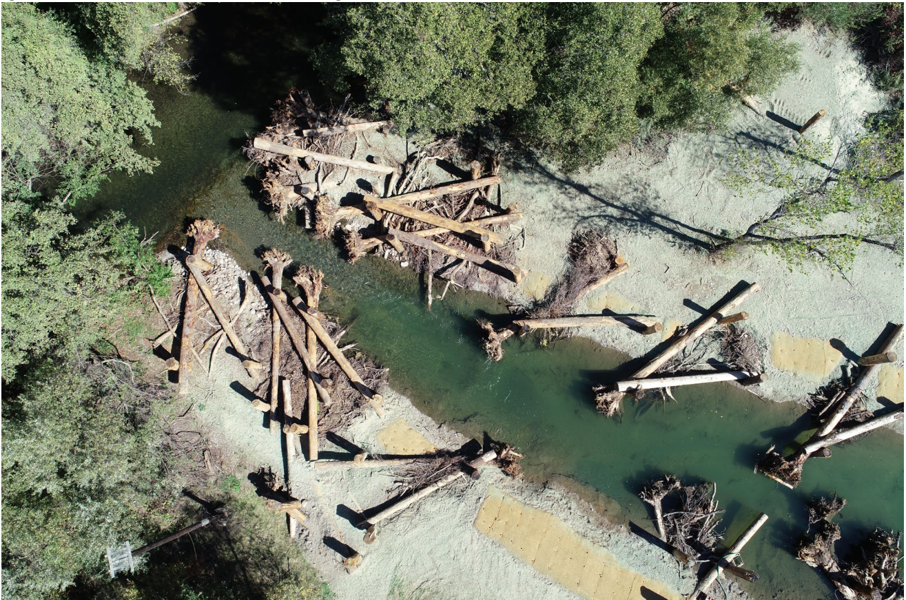
Site Progression Monitoring Photo. Reach 14 site at completion of construction. Photo shows a portion of the completed side channel. Photo taken October 10, 2018.
