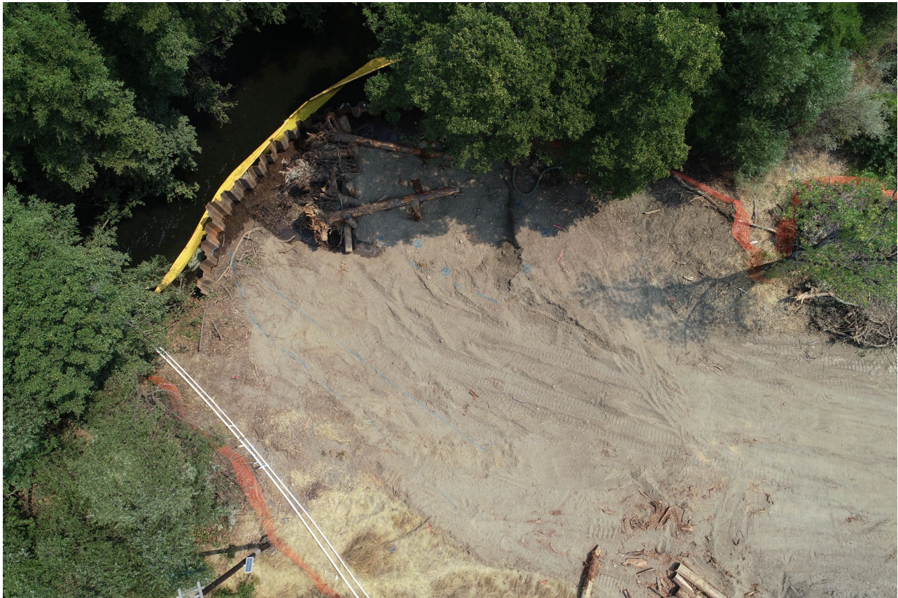
Site Progression Monitoring Photo. Reach 14 site during construction. Photo showing sheet pile installed to isolate construction area from mainstem of Dry Creek and the start of earthwork and log installation. Photo taken August 8, 2018.
