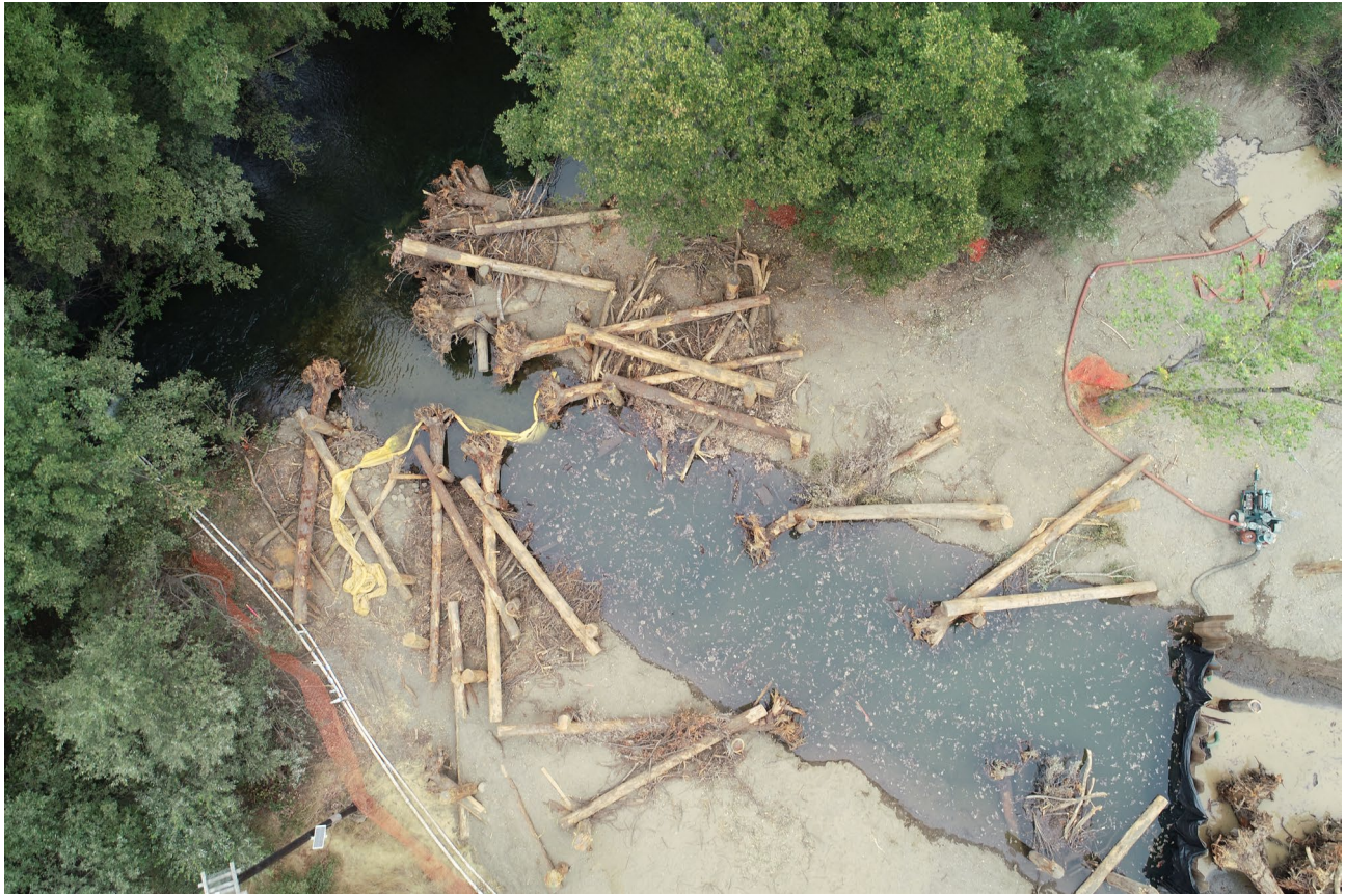
Site Progression Monitoring Photo. Reach 14 site during construction. Photo showing sheet pile moved further into the constructed side channel to isolate the construction work area. Photo also shows the further progression of earthwork and log structure installation. Photo taken August 23, 2018.
