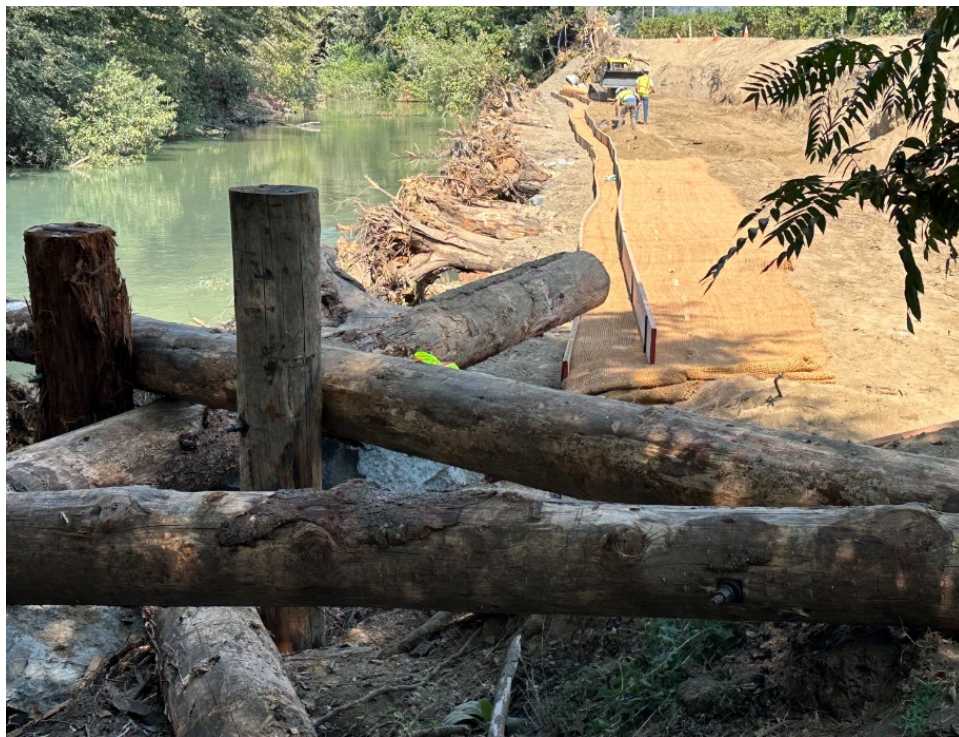
Photograph taken on September 19, 2023 of construction of a biotechnical bank repair and habitat enhancement in Reach 10 of Dry Creek.
