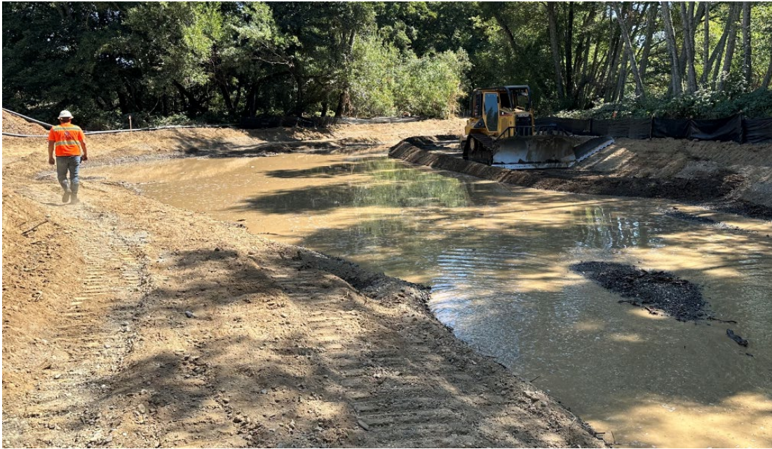
Photograph taken on 9/13/23 showing partially excavated new side-channel habitat feature at site 4C.
