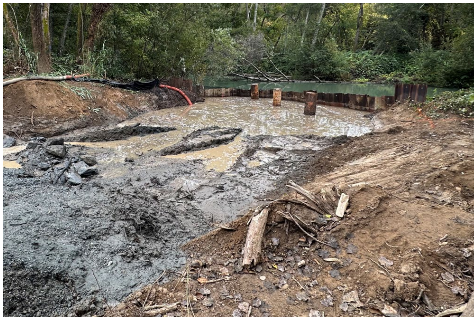
Photograph taken on 10/25/23 showing partially completed inlet to the new side-channel habitat feature at site 4C.
