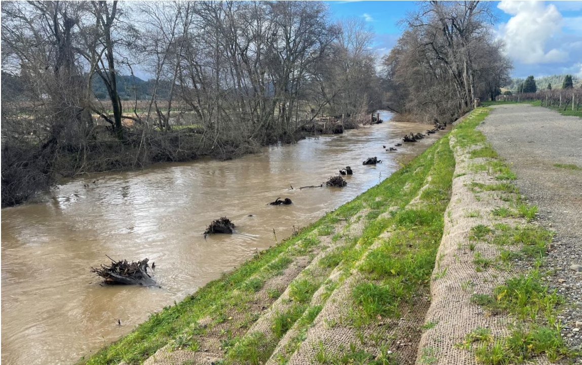
Photograph taken during the high flow event on January 22, 2024 of the upstream end of a completed Reach 10 biotechnical bank repair.
