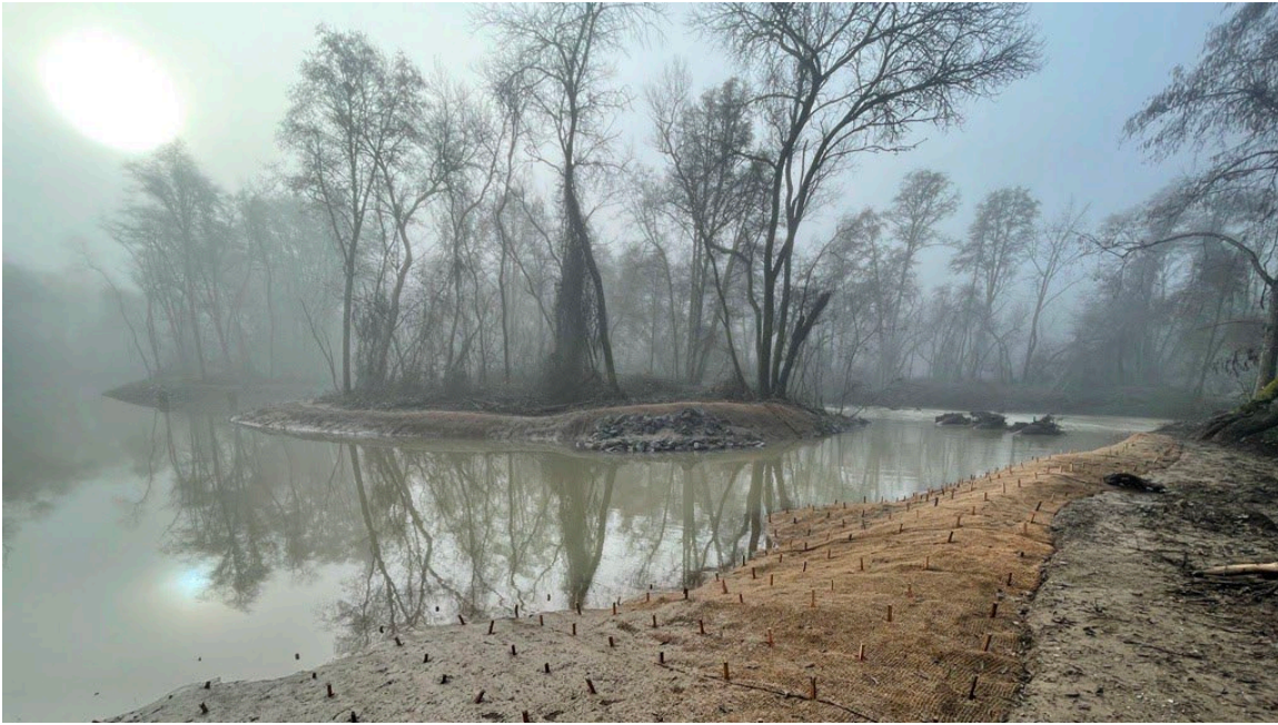
Photograph taken on January 23, 2024 showing one of the intermediate inlets to the new side-channel habitat feature at site 4C at a flow of approximately 800 cfs.
