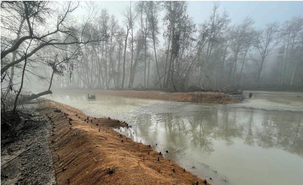
Photograph taken on January 23, 2024 showing one of the intermediate inlets to the new side-channel habitat feature at site 4C at a flow of approximately 800 cfs.
