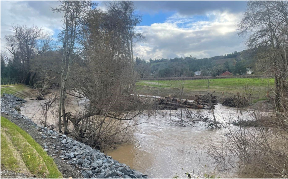
Photograph taken on January 22, 2024 of the 10A0 bank repair and high-flow side channel.
