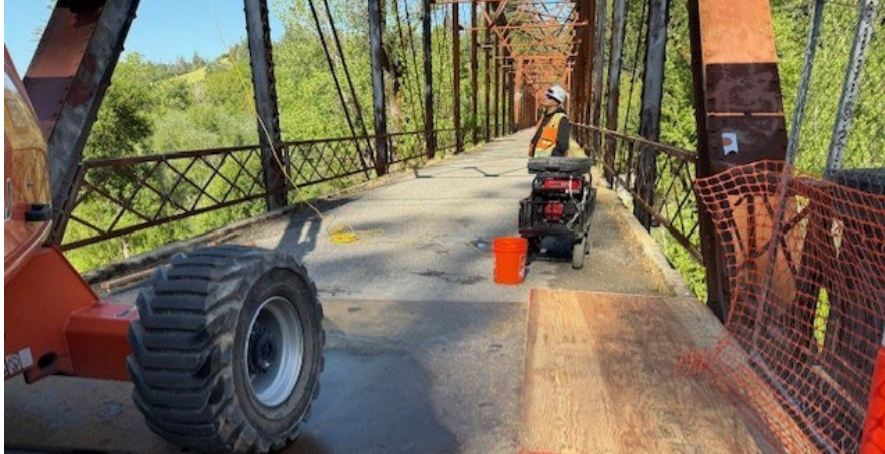
Wohler Bridge Seismic Retrofit
