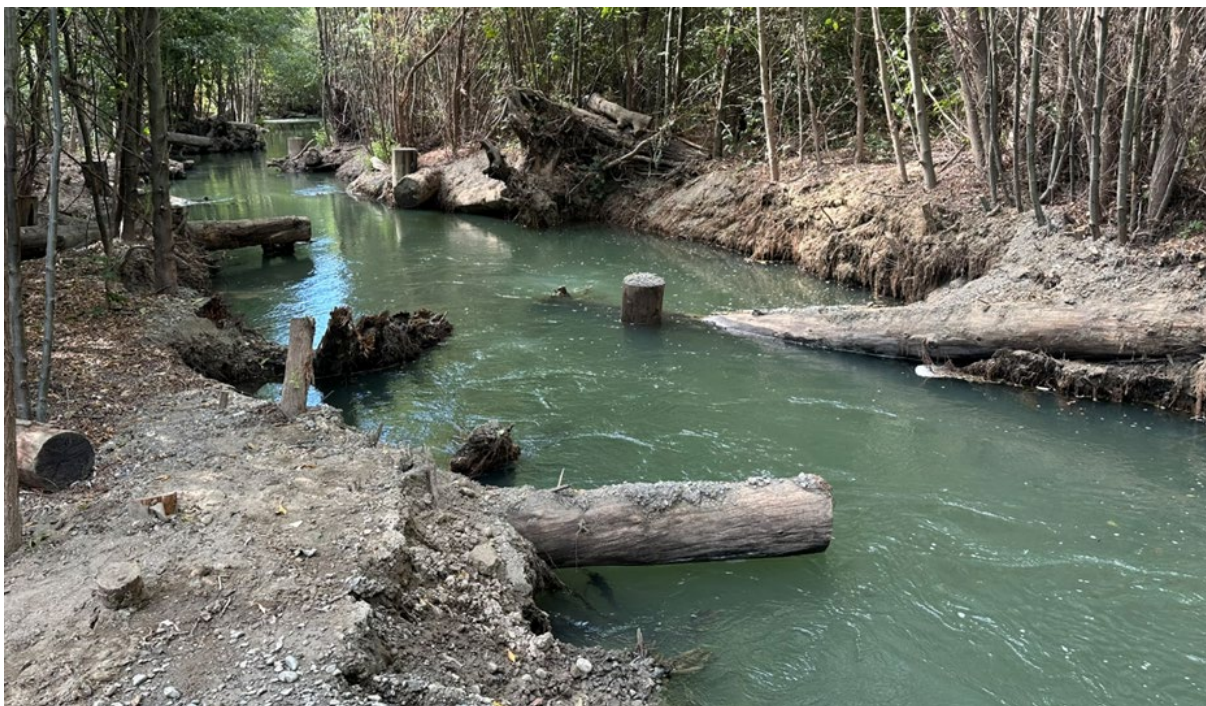
Free-flowing condition of the site 8d side channel after sediment removal.
