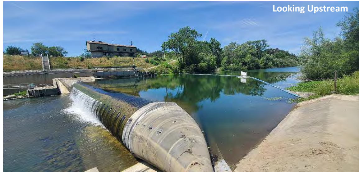
Mirabel Inlatable Dam
