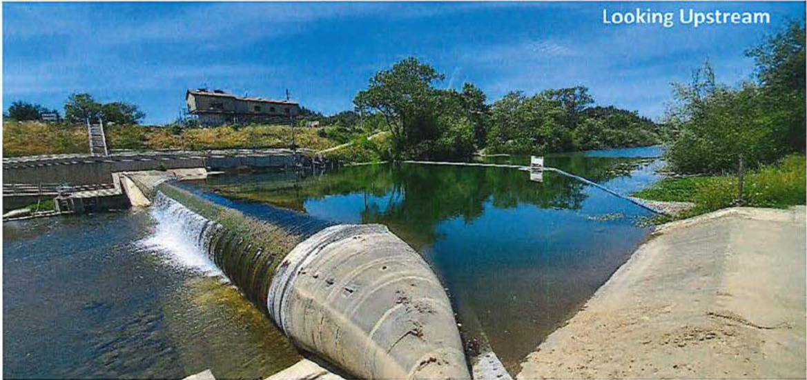
Mirabel Inflatable Dam
