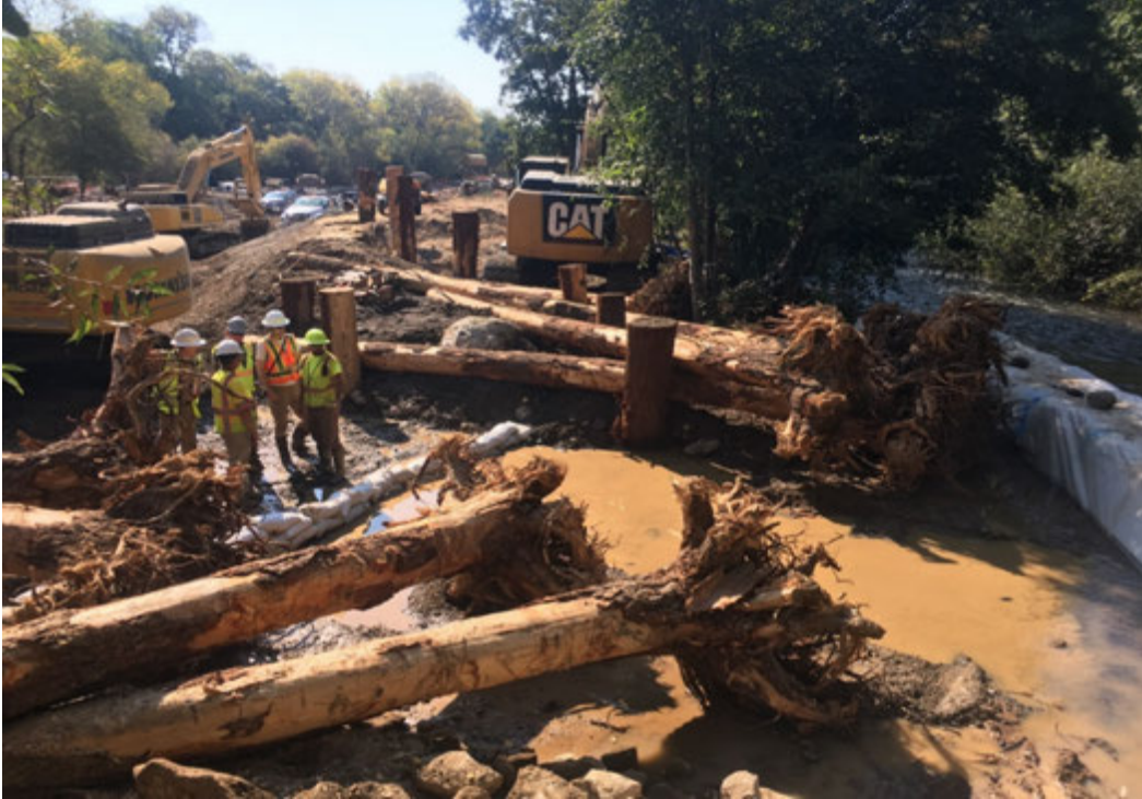
Photo 5.1.1. Dry Creek Habitat Enhancement Project Phase 2, Part 1. Photo shows new side channel inlet under construction at the Truett Hurst site (Reach 8). Mainstem of Dry Creek (looking downstream) can be seen at the right hand side of the photo. August 2016.
