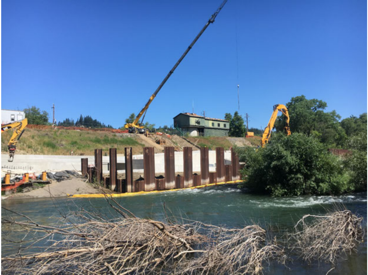
Photo 8. 5. The sheet pile in place since 2014 for isolating the job site from the Russian River is being removed. May 21, 2016.
