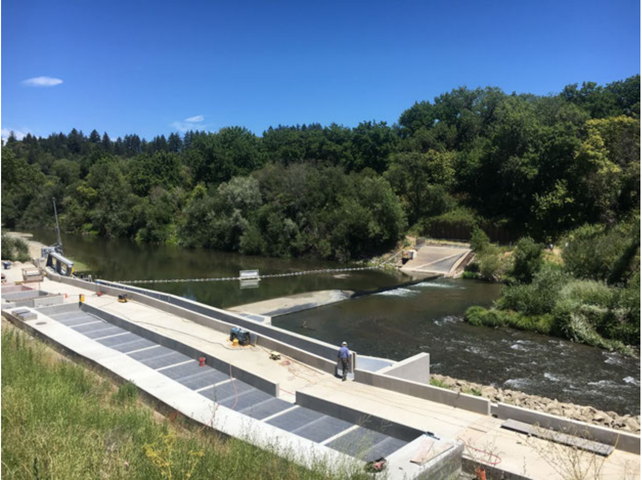
Photo 8. 8. The Mirabel inflatable dam being raised again. July 8, 2016.
