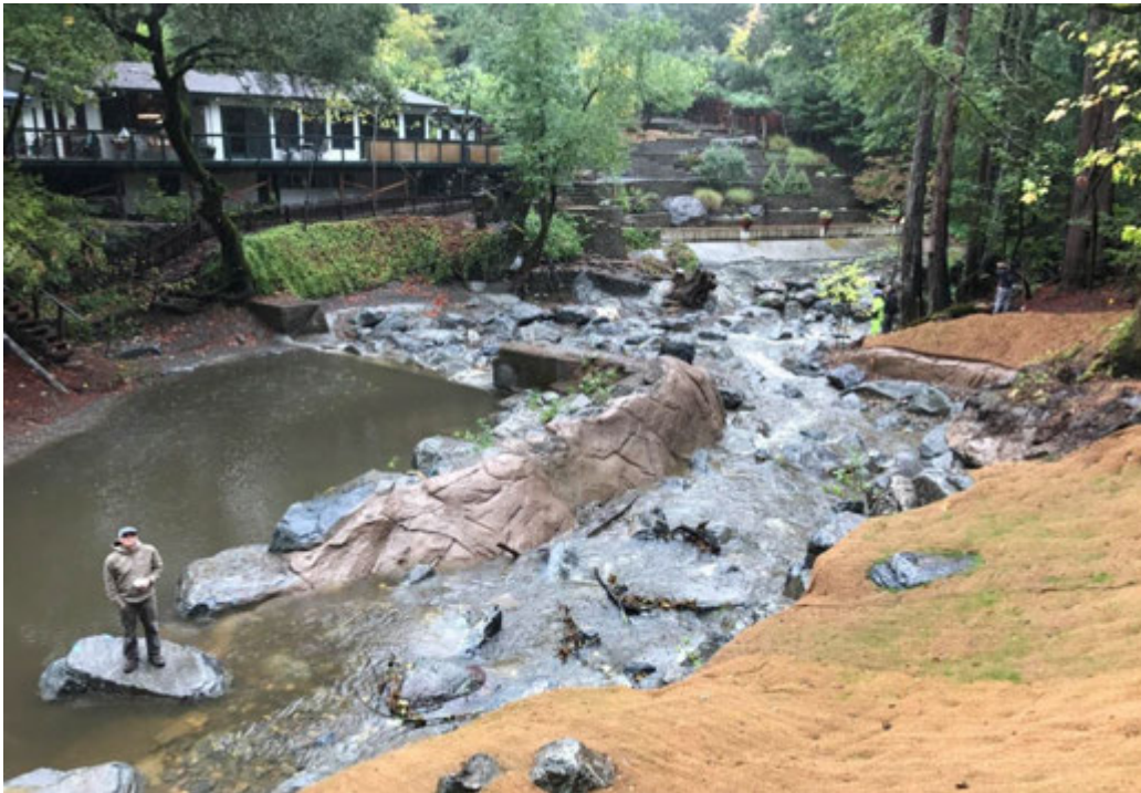
Figure 6. 17. Mill Creek Fish Passage Project. Showing completed new bypass channel and roughened ramp on downstream side of the passage barrier in Mill Creek. October 2016.
