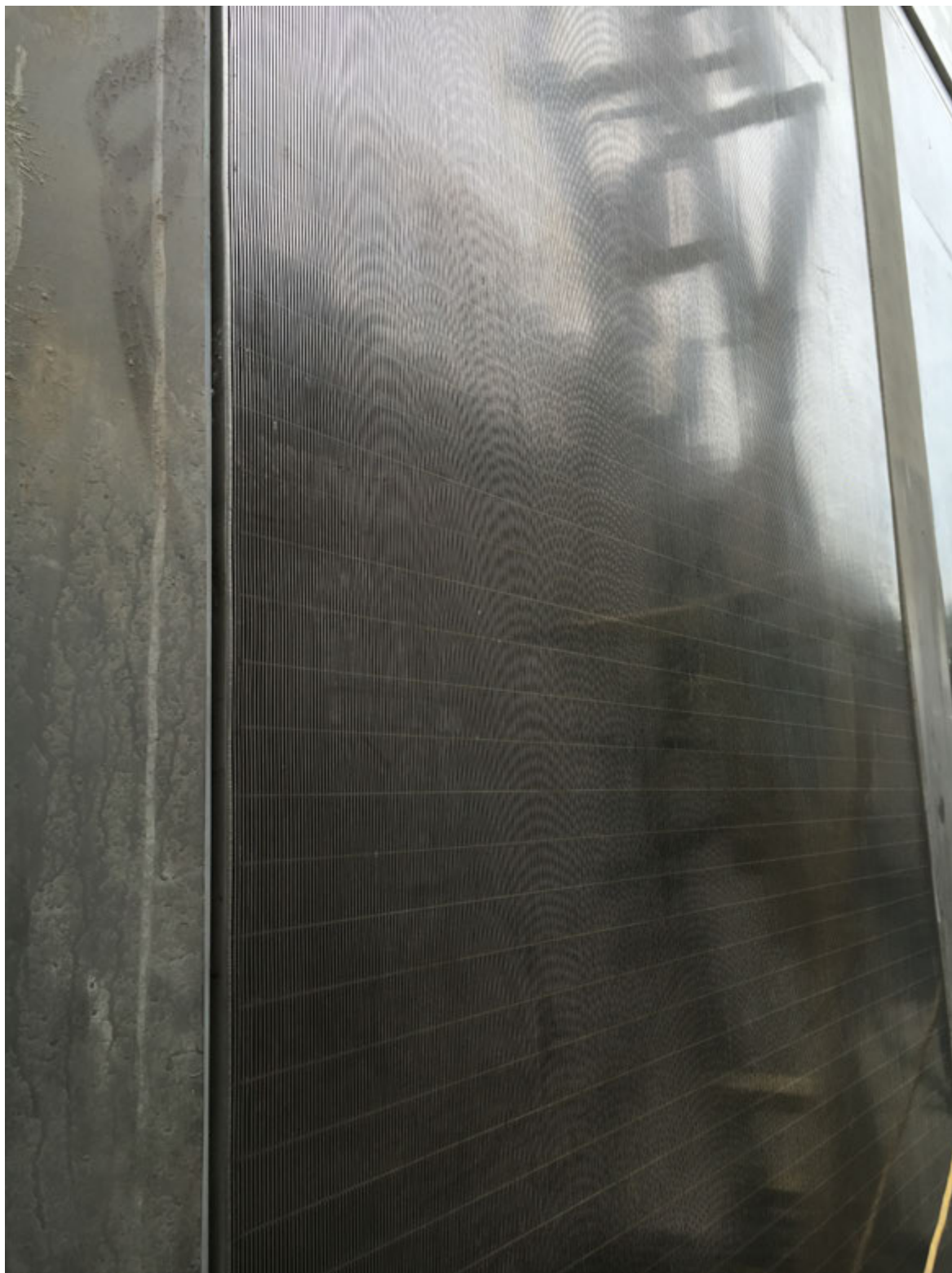
Photo 8. 3. The new flat-panel diversion screens are in place. May 4, 2016.
