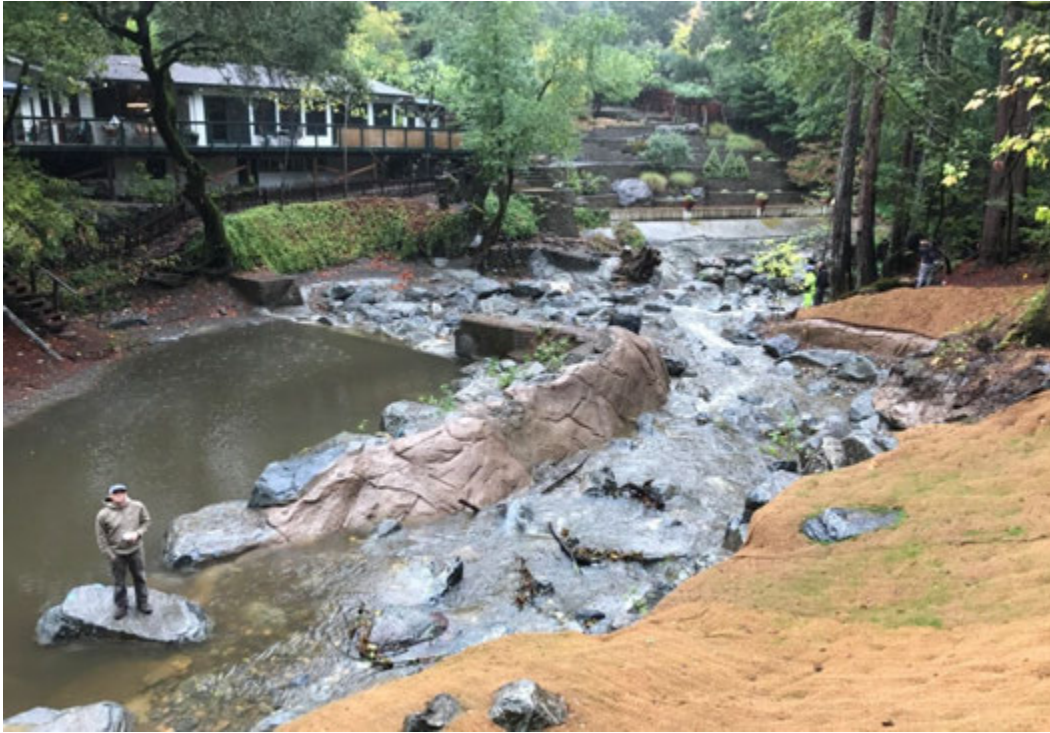
Figure 1. View of Mill Creek Dam Fish Passage Project less than one month after construction completion (looking downstream). Constructed side channel with 3% slope is in the foreground with pre-existing dam and the main channel roughened ramp in center of photo.
