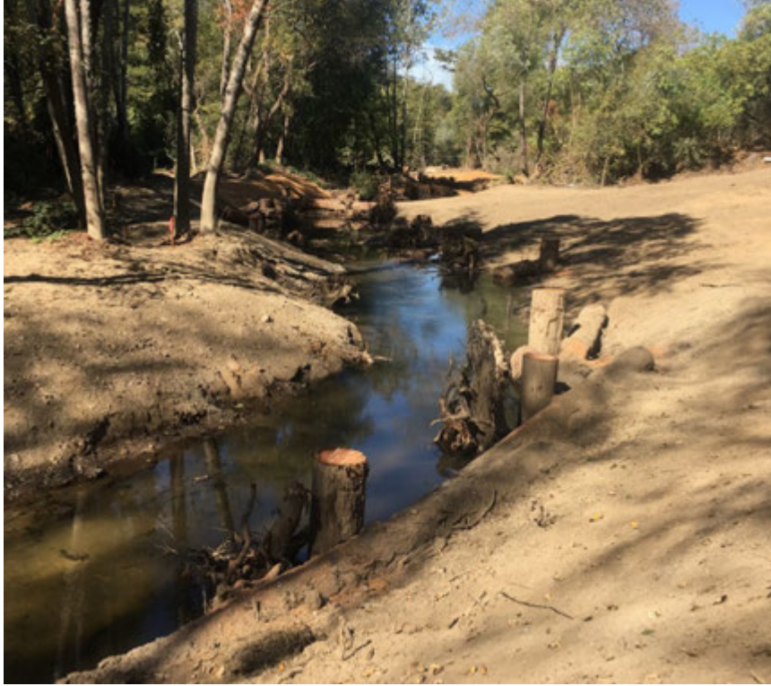
Photo 5.1.3. Dry Creek Habitat Enhancement Project Phase 3, Part 1. New side channel feature recently constructed at the Geyser Peak site (Reach 2). October 2016.
