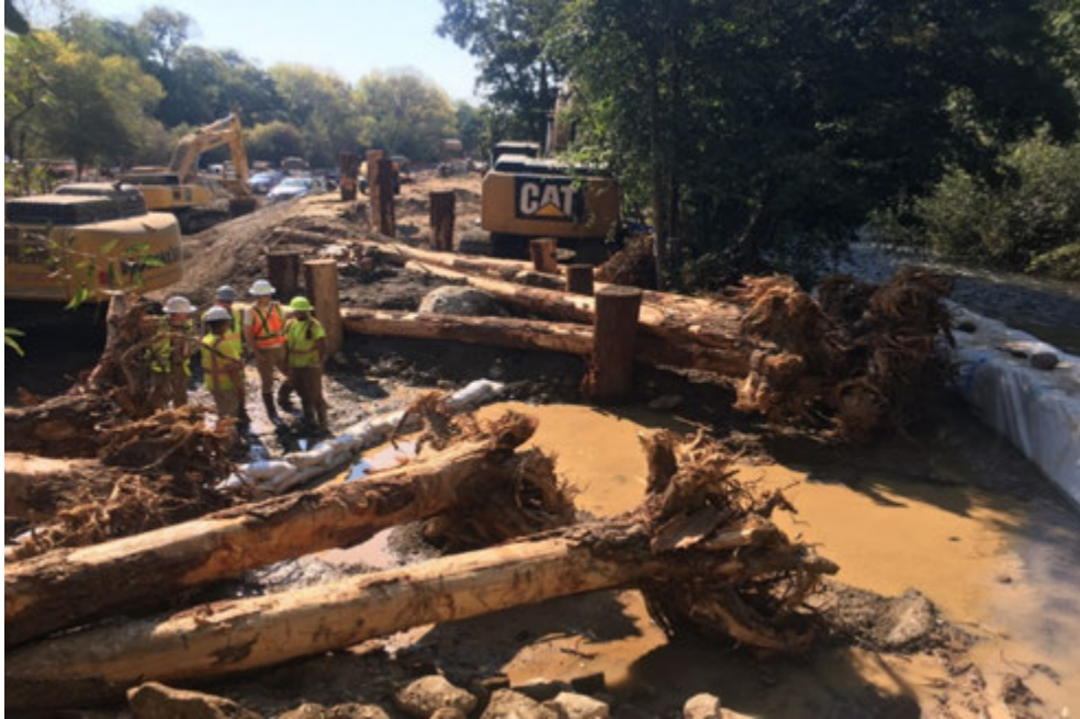
Photo 5.1.1. Dry Creek Habitat Enhancement Project Phase 2, Part 1. New side channel inlet under construction at the Truett Hurst site (Reach 8). Mainstem of Dry Creek (looking downstream) can be seen at the right hand side of the photo. August 2016.
