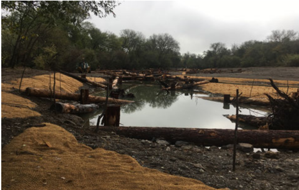
Photo 5.1.2. Dry Creek Habitat Enhancement Project Phase 2, Part 1. New side channel backwater feature recently constructed at the Truett Hurst site (Reach 8). October 2016.
