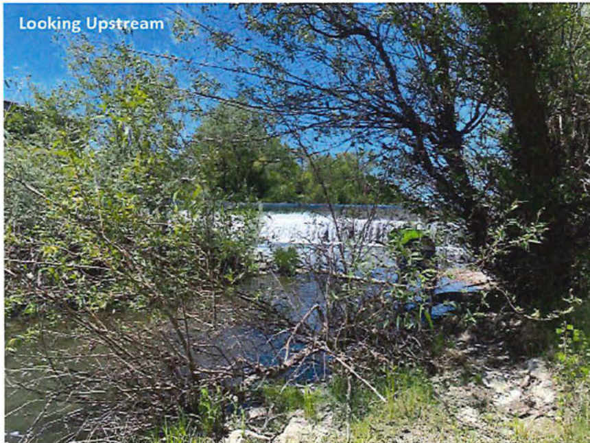
Mirabel Inflatable Dam
