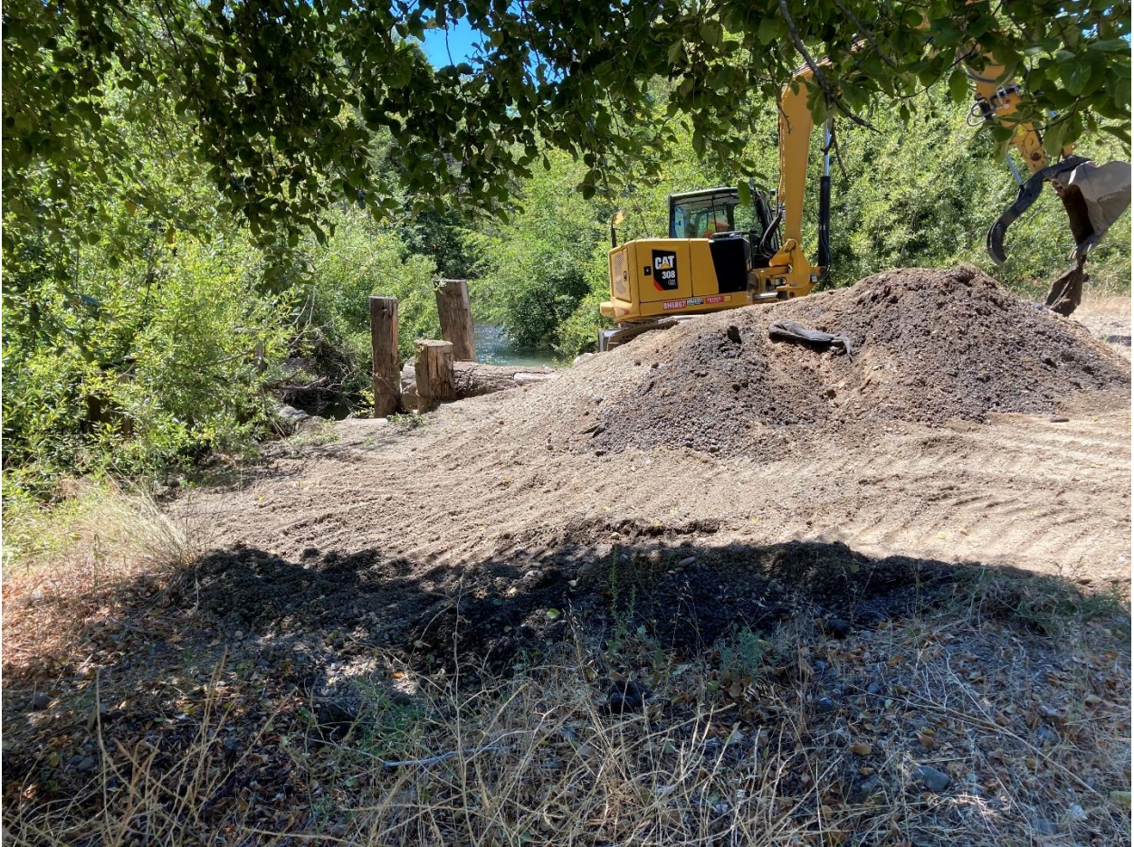
Photo 5.1.22. Reach 7 - Farrow site. Start of erosion repair work. July 30, 2020.
