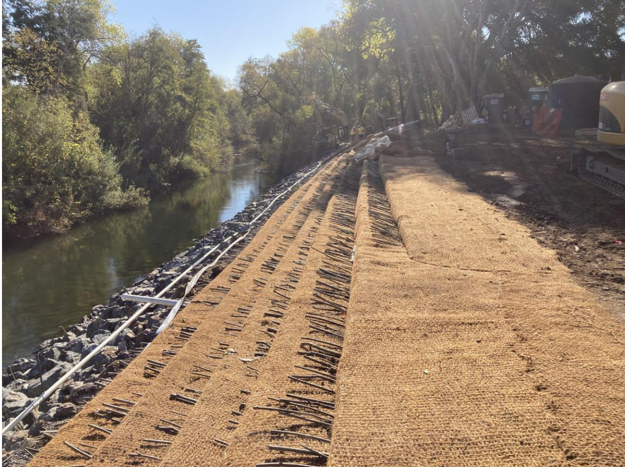
Photo 5.1.7. Phase 3, Part 3. Bank stabilization section work is complete. November 3, 2020.
