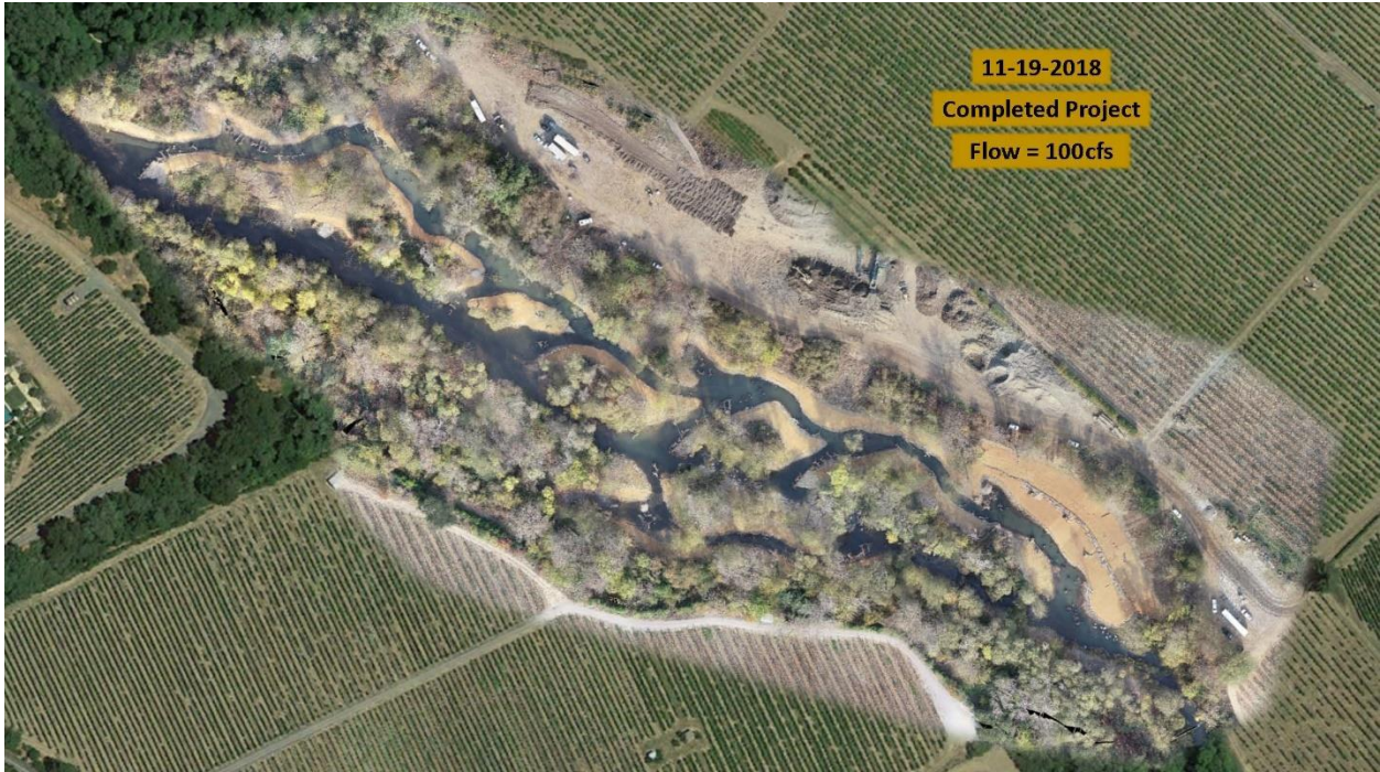
Photo 5.1.8. Reach 4A Site Post-Construction on November 19, 2018.
