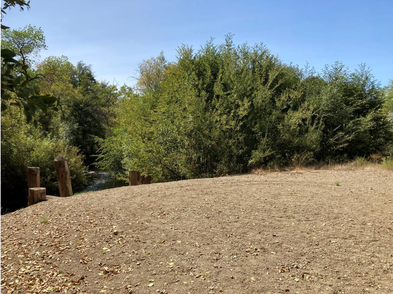
Photo 5.1.25. Reach 7 - Farrow site. Completed erosion repair at engineered logjam. September 17, 2020.
