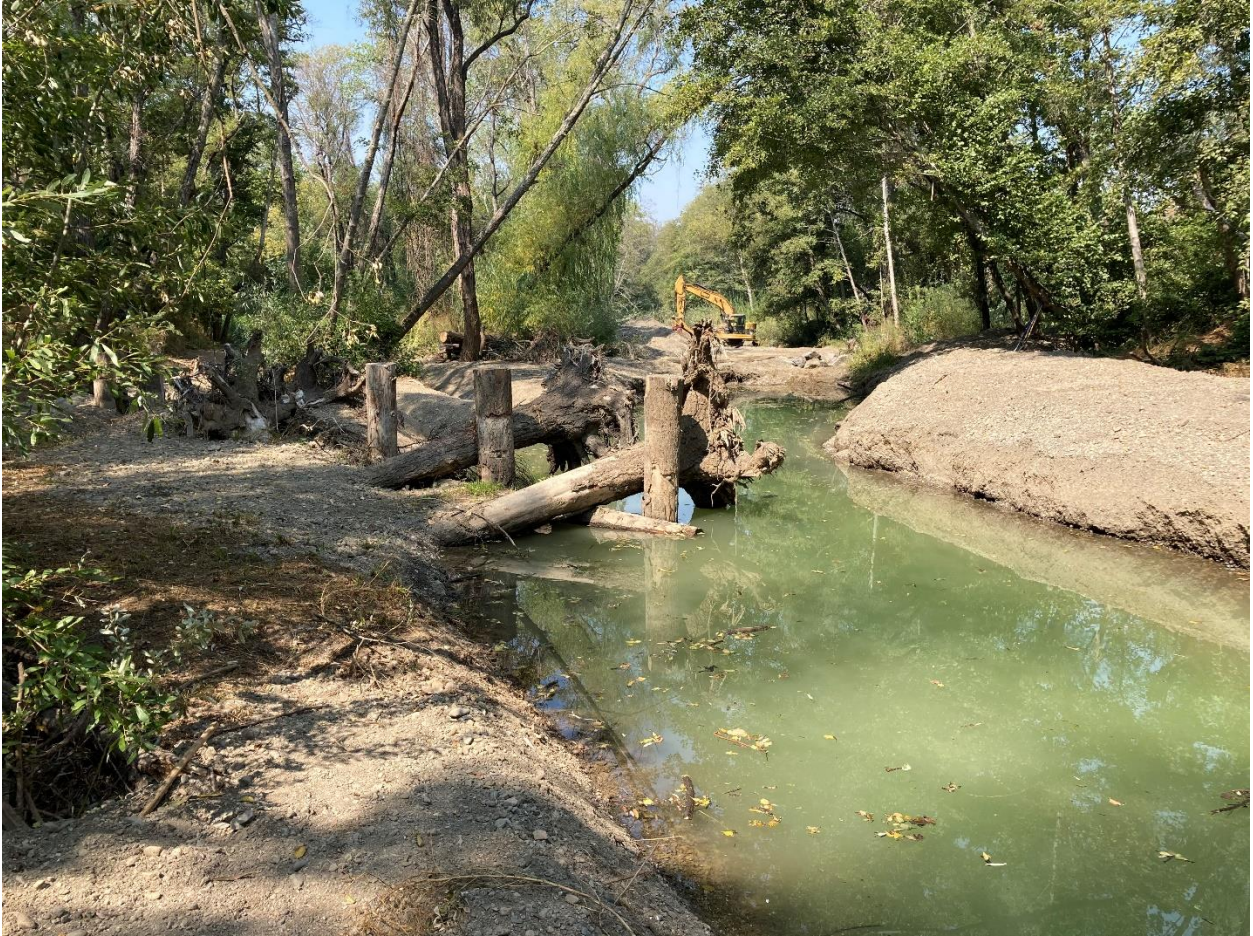
Photo 5.1.17. Reach 4A. Same view as in photo 5.1.10 above. Low flow channel re-established and existing habitat structure exposed again. September 21, 2020.
