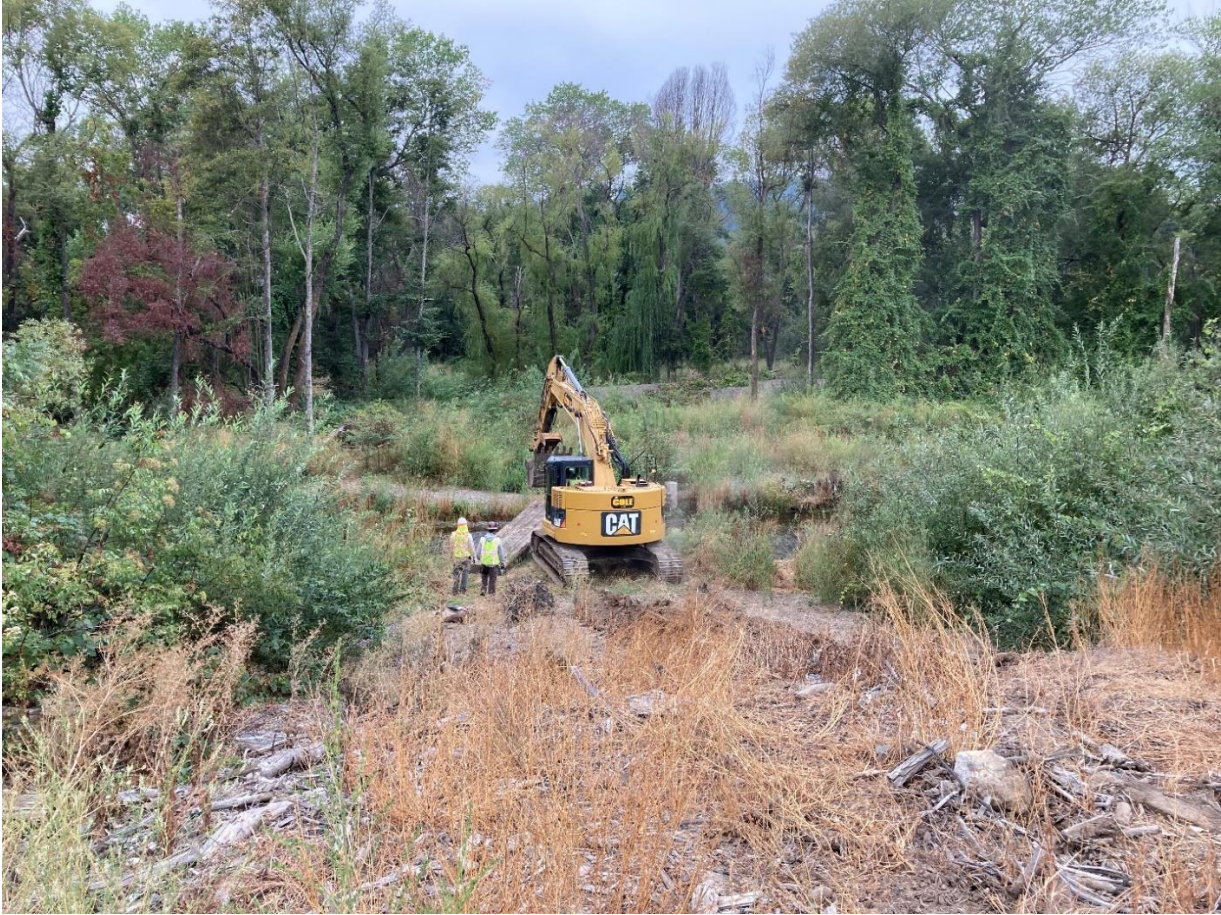
Photo 5.1.14. Reach 4A. Bridge crossing installation. September 2, 2020.
