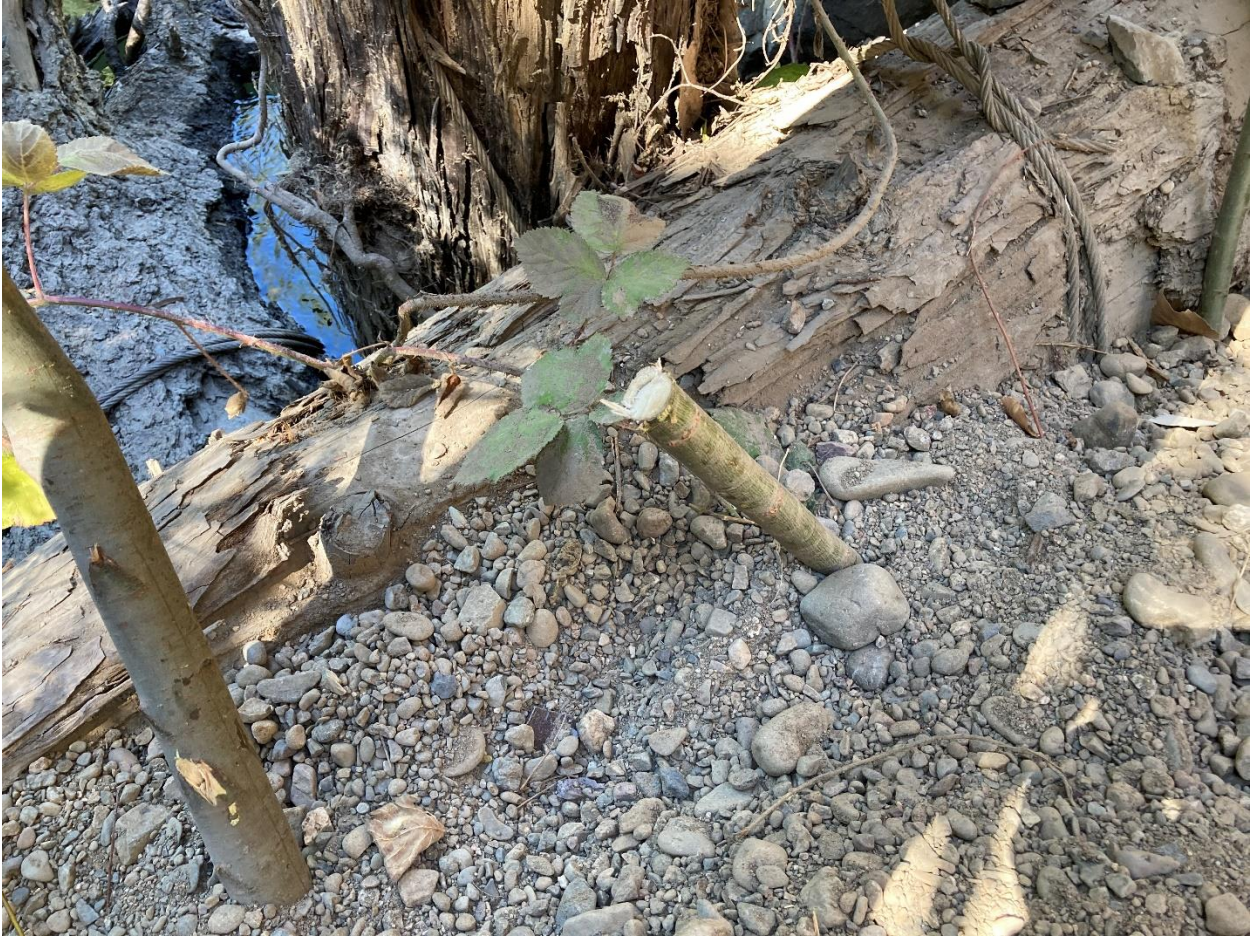
Photo 5.1.23. Reach 7 - Farrow site. New willow cuttings installed in engineered logjam. August 4, 2020.
