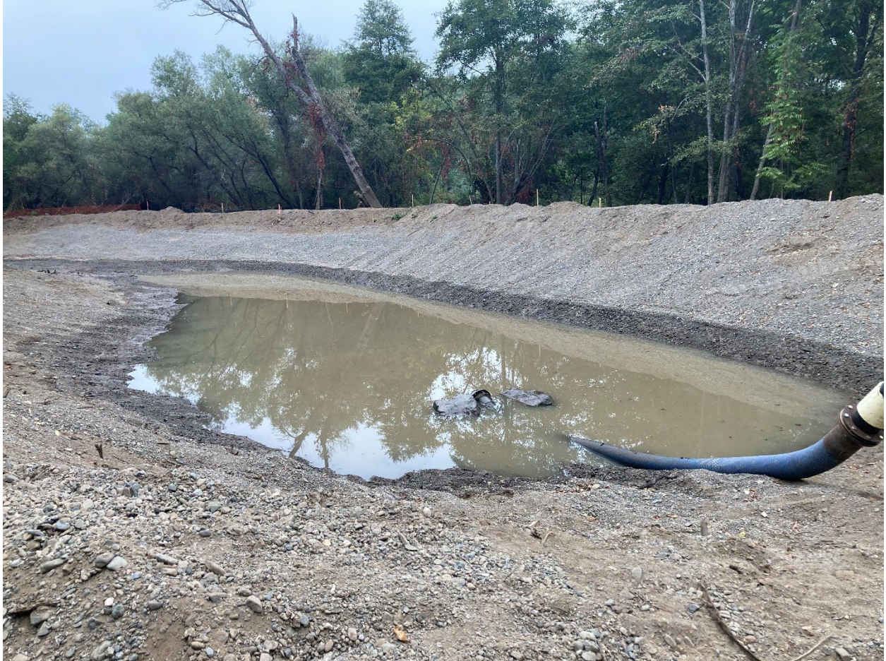
Photo 5.1.6. Phase 3, Part 3. Initial clearing of habitat site work area and being used as a dewatering basin for the bank stabilization work. September 10, 2020.
