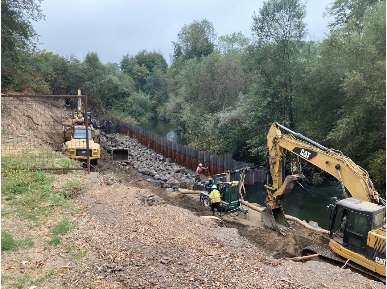
Photo 5.1.5. Phase 3, Part 3. Rock slope protection construction in progress. Note sheet-pile isolating work area from active flow of Dry Creek. September 10, 2020.
