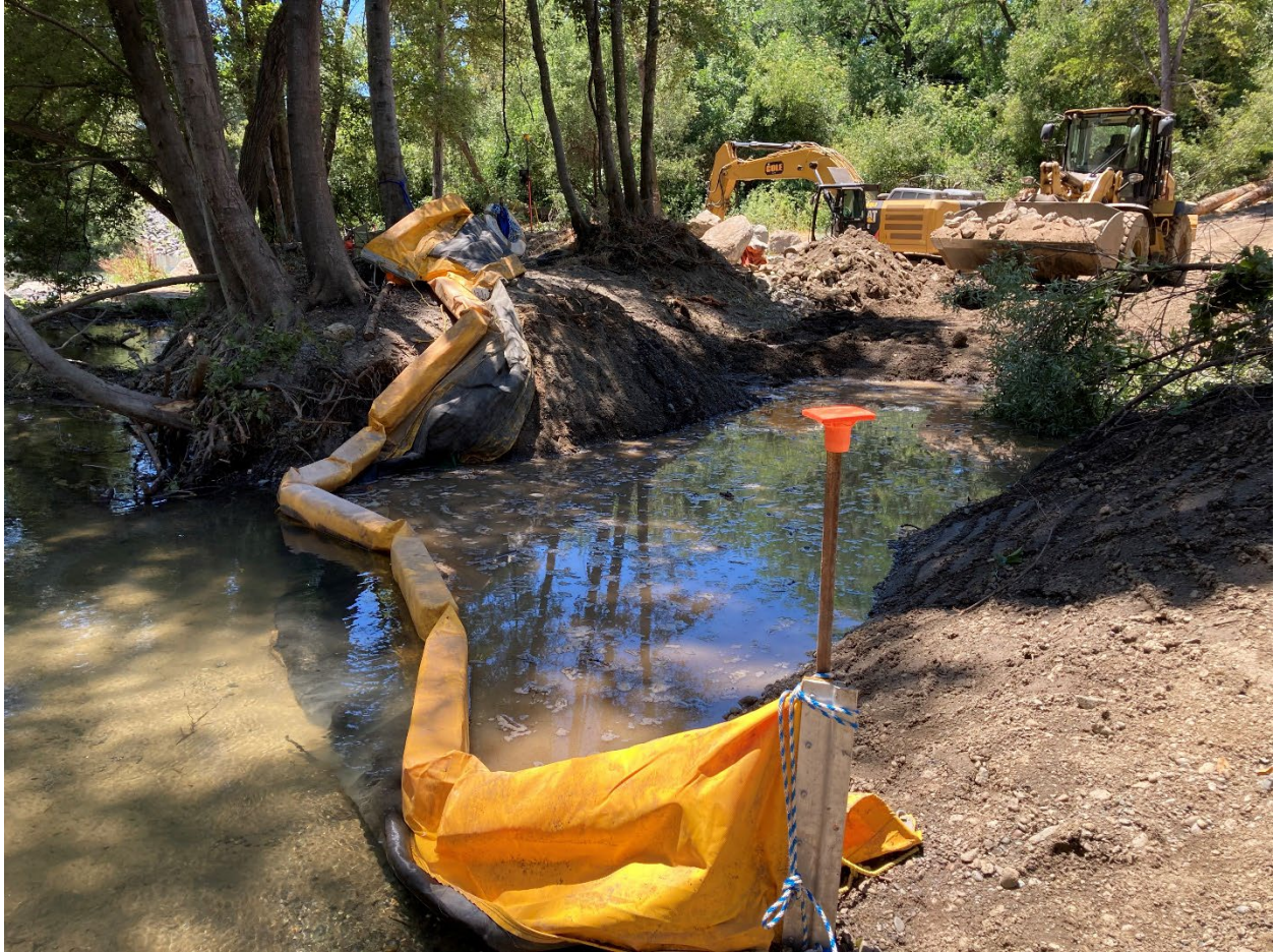
Photo 5.1.10. Phase 3, Part 3. New habitat side-channel feature under construction (Stromberg site). Photo is showing the side-channel inlet area with a turbidity curtain isolating the inlet area from the active flow of Dry Creek. June 24, 2021.
