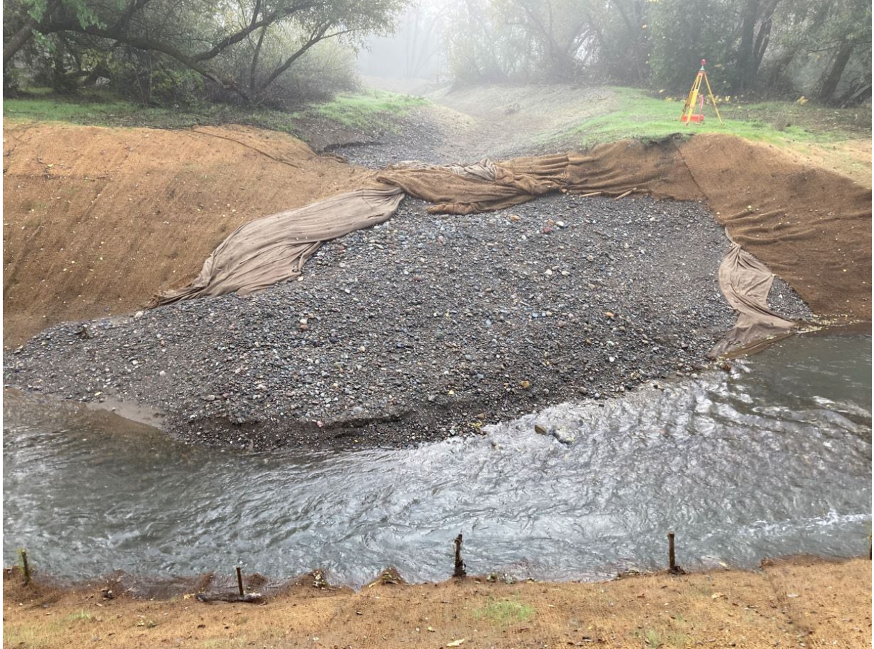
Photo 5.1.17. Phase 3, Part 3. Minor damage to erosion control fabric in the inlet area to the Gros-Balthazard site side channel as a result of the October 24, 2021 high flow event. November 3, 2021.
