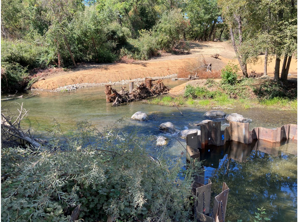
Photo 5.1.11. Phase 3, Part 3. New habitat side-channel feature (Stromberg site) recently completed, showing the side-channel outlet back into the mainstem of Dry Creek. Also visible in this photo is a newly installed boulder field in the mainstem of Dry Creek, and a portion of sheet piling being used to isolate the active flow of Dry Creek from the Gros-Balthazard site work area). August 25, 2021.
