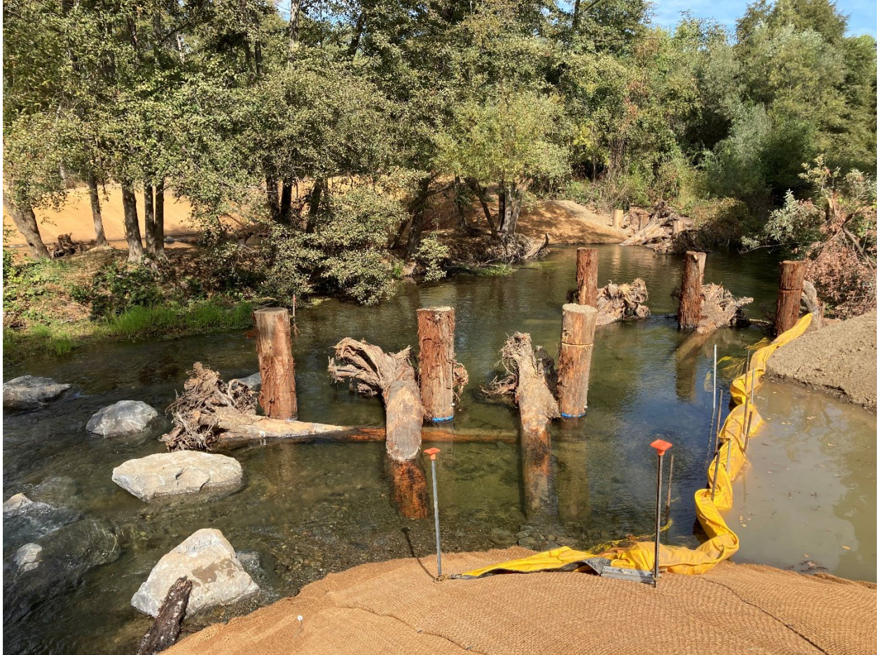
Photo 5.1.14. Phase 3, Part 3. Newly installed wood structures at the inlet to the habitat side-channel feature (Gros-Balthazard site). The side-channel is under construction and a turbidity curtain is visible isolating the work area from the active flow of Dry Creek. September 8, 2021.
