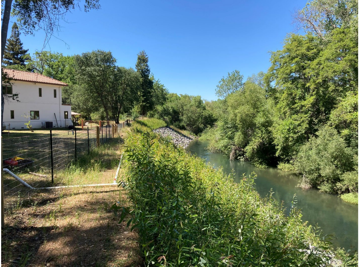
Photo 5.1.9. Phase 3, Part 3. Bank stabilization section work completed in 2020 and showing willow cuttings established and leafing out. May 19, 2021.
