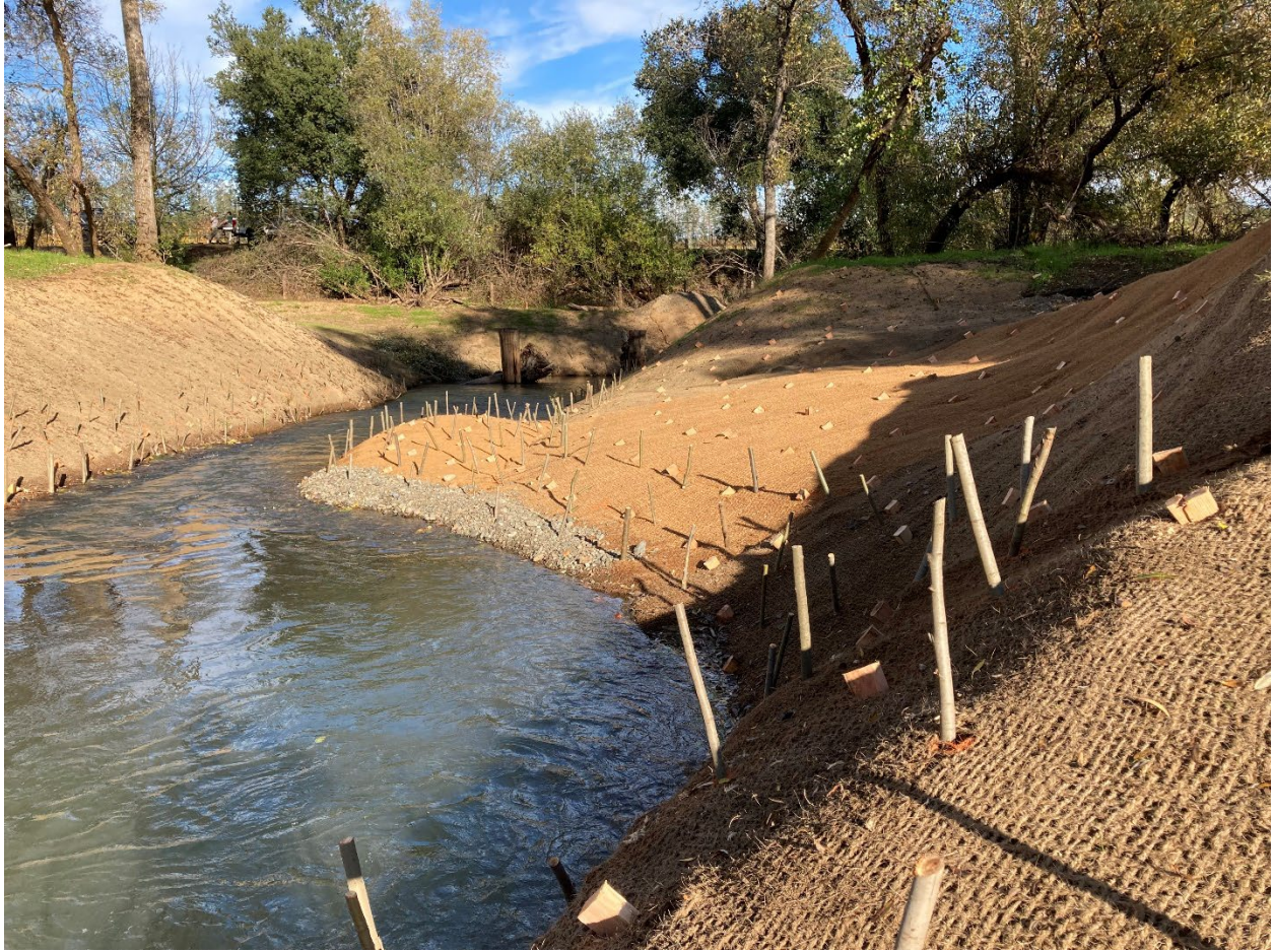
Photo 5.1.18. Phase 3, Part 3. Inlet area to the Gros-Balthazard, erosion control fabric repaired and area re-staked with willow cuttings after the October 24, 2021 high flow event. November 23, 2021.
