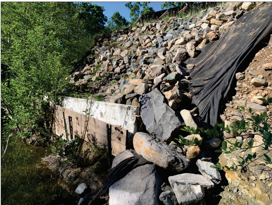
Figure 10. Temporary riprap eroded/moved at upstream end exposing underlying geogrid filter fabric during series of atmospheric rivers. K-rail is also undermined and supported primarily by three steel rods installed in fall 2022. (Photo by SVCSD May 2023)
