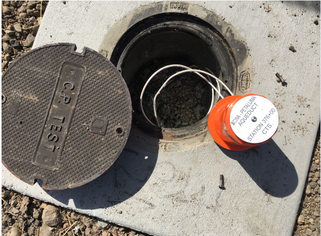
Figure 2-27. Finished flush-mounted test station.
