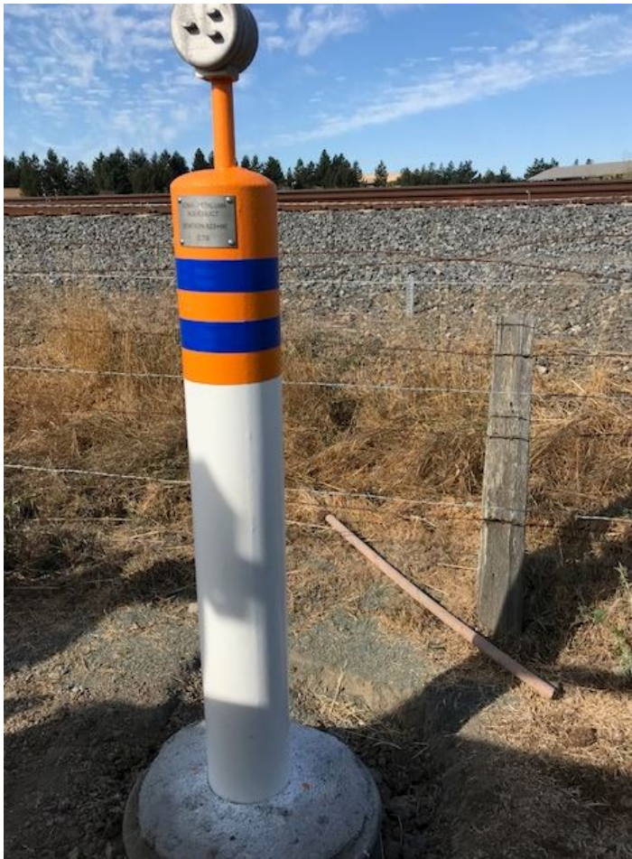
Figure 2-25. Aboveground components of a test station may include a four-foot post with a small test box at the top.
