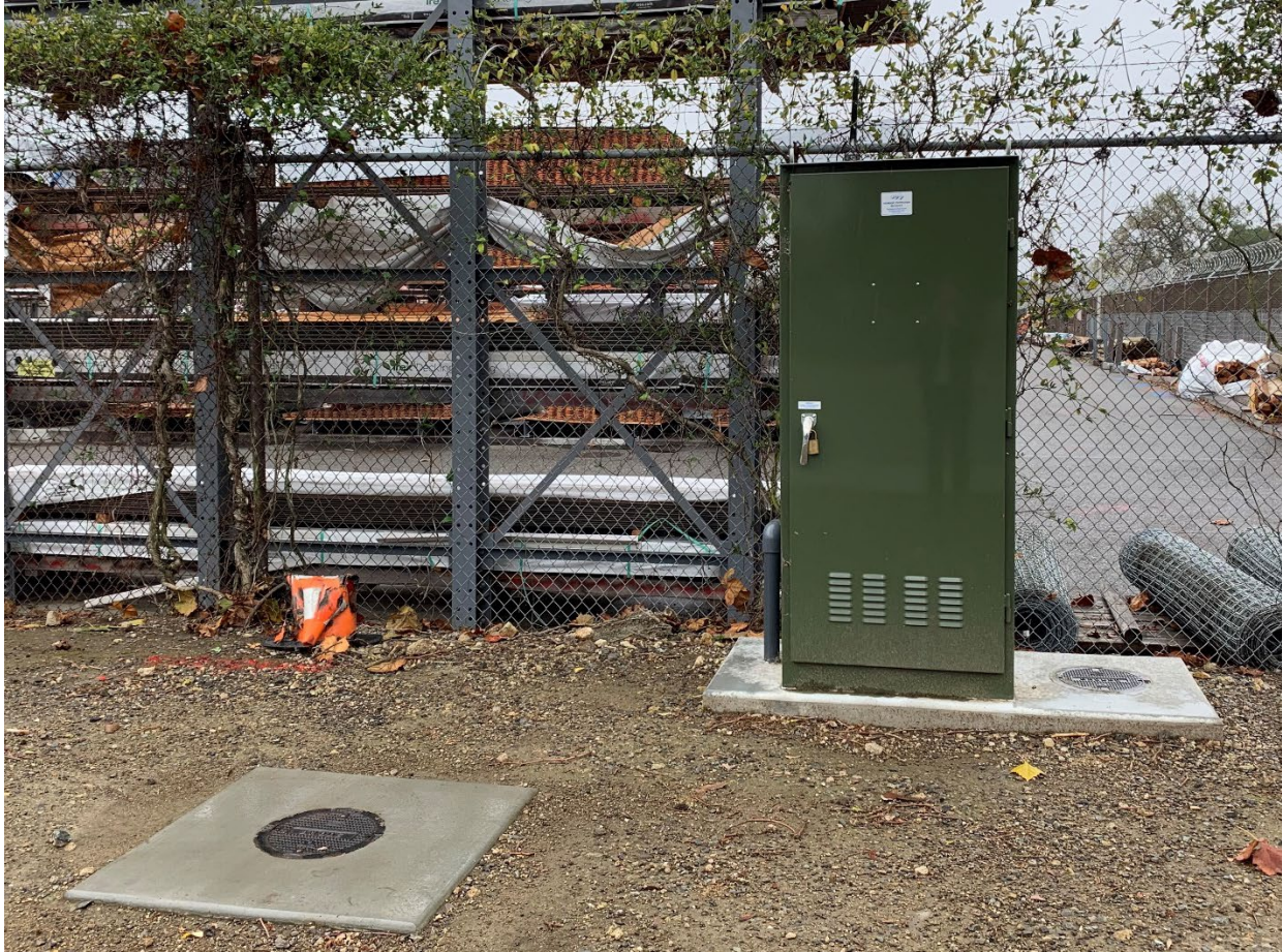
Figure 2-23. Visible aboveground components of a Cathodic Protection Station. These would include an olive-green cabinet housing the rectifier (above, right), which would measure approximately three feet wide and five feet tall, and the cap of the anode well (above, left). Two of the proposed sites would include a solar array measuring approximately ten feet by fifteen feet in place of a rectifier cabinet.
