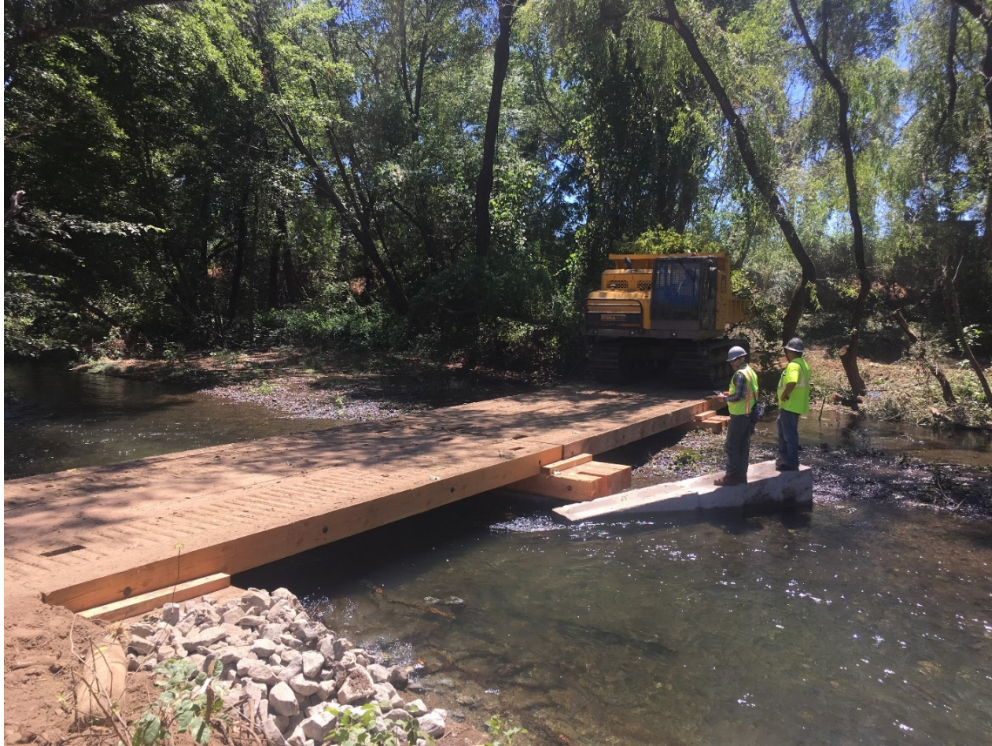
Photo 5.1.5. Dry Creek Enhancement Project Phase 3, Part 2, Ferrari-Carano, Olson, temporary crossing of Dry Creek during construction. July 26, 2018.
