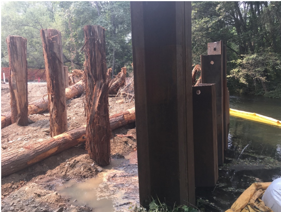
Photo 5.1.2. Dry Creek Enhancement Project Phase 2, Part 2, Army Corps Reach 14 (Area J) upstream inlet under construction. Installed logs visible on the left, sheet pile isolating the work area from Dry Creek is visible in the center of the photo, and the active flow of Dry Creek is on the right. August 7, 2018.
