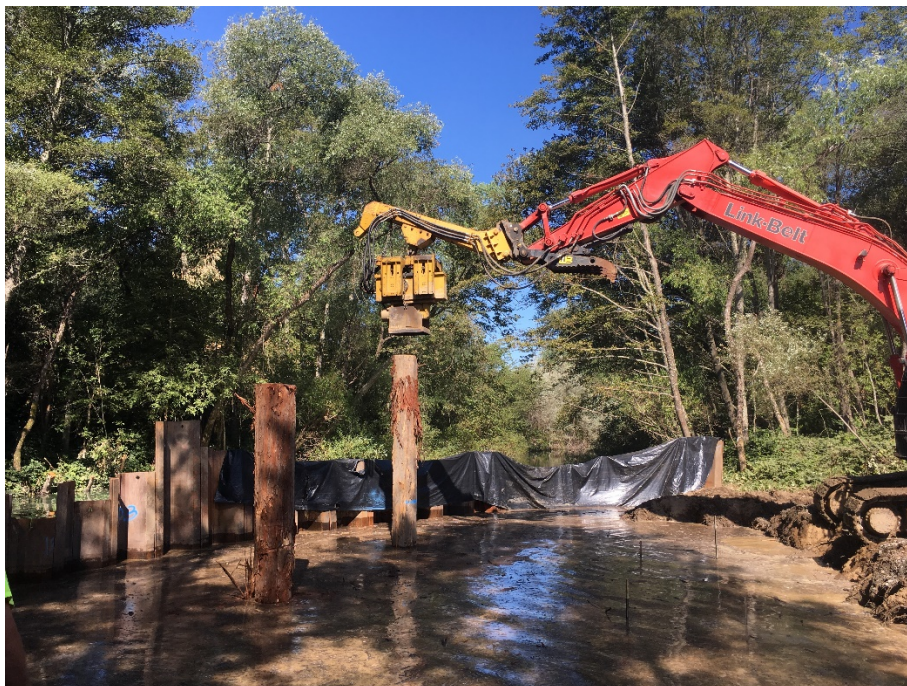
Photo 5.1.4. Phase 2, Part 2, Area G. Driving vertical snags for the log structure at the upper inlet to the site. Note sheet pile in place isolating the turbid water of the work area from the mainstem of Dry Creek. July 31, 2019.
