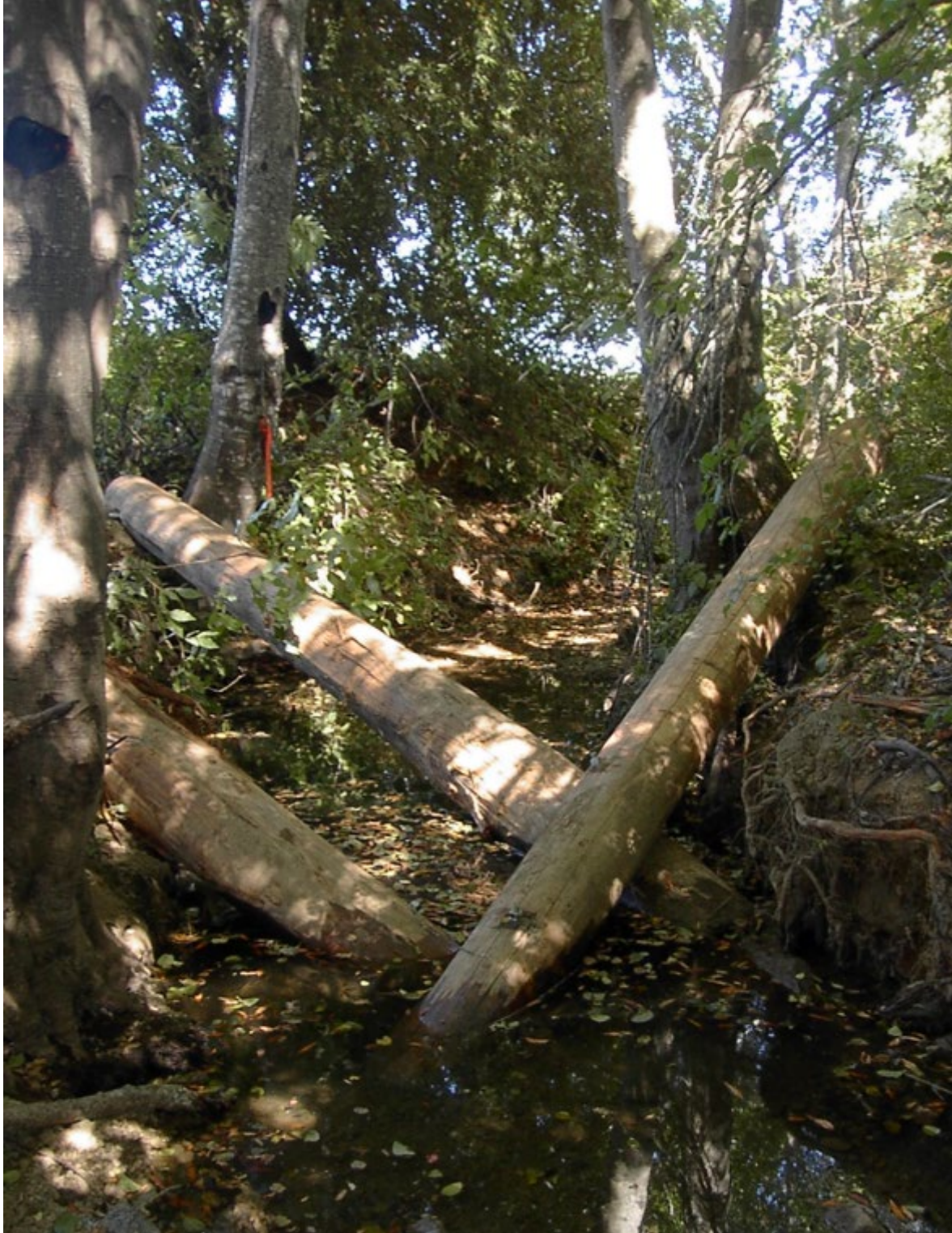
Figure 6. 1. Grape Creek – Phase 1. In-Stream Large Woody Debris Structure Example (2009 post construction).
