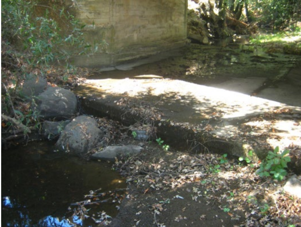
Figure 6. 13. Grape Creek Fish Passage Project – Flat culvert invert proposed for modification.
