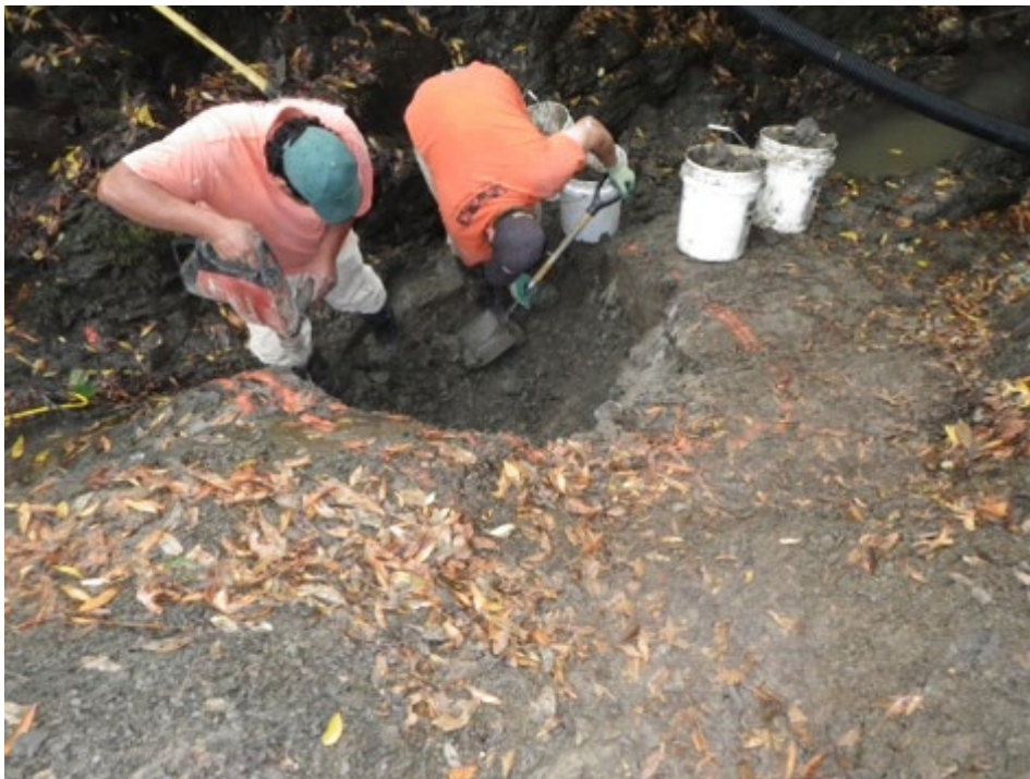
Figure 6. 11. Crane Creek Fish Passage Access Project. Chiseling pools in bedrock outcropping.
