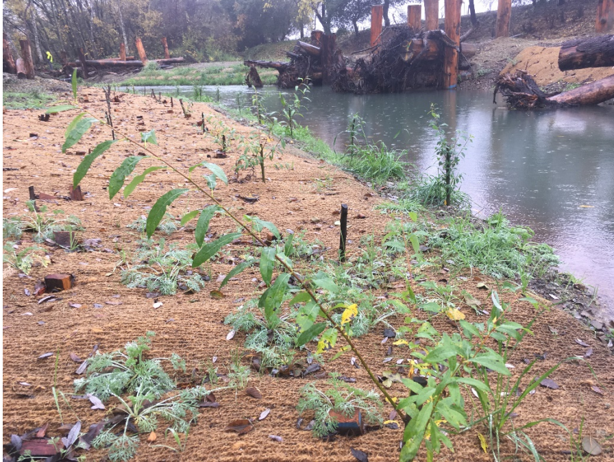
Photo 5.1.7. Phase 2, Part 2, Area G. Construction of new side channel is complete. Installed willow cuttings have started to leaf out. View is looking upstream towards the upper inlet. December 11, 2019.
