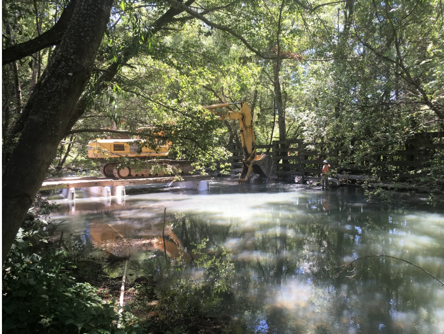
Photo 5.1.5. Phase 2, Part 2, Area G. Installation of boulder field in mainstem of Dry Creek. Note temporary bridge installed to keep excavator tracks out of the active flow while boulders are placed. July 22, 2019.
