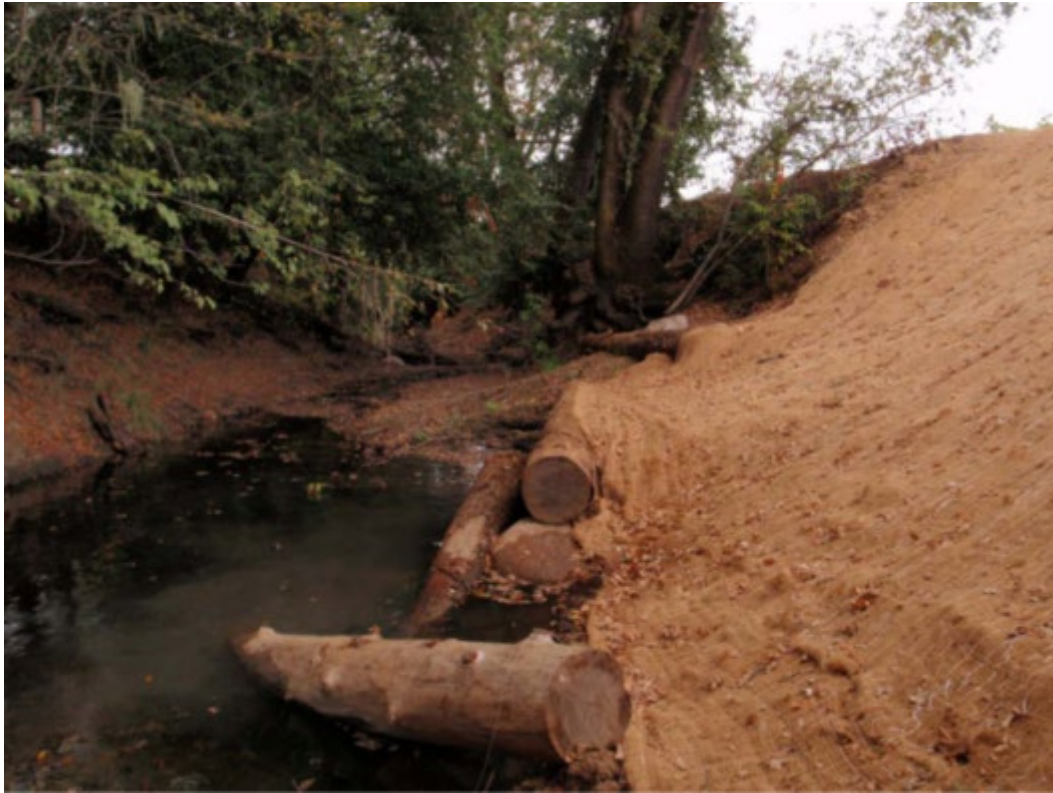
Figure 6. 5. Grape Creek – Phase 2. Large Woody Debris and Bank Layback Example.
