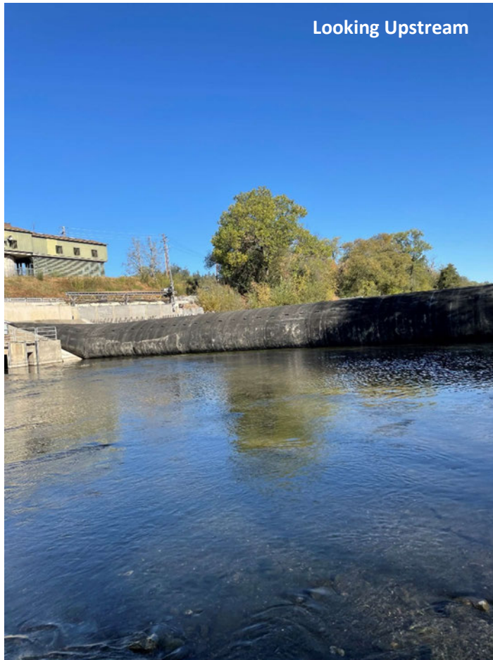
Mirabel Inflatable Dam
