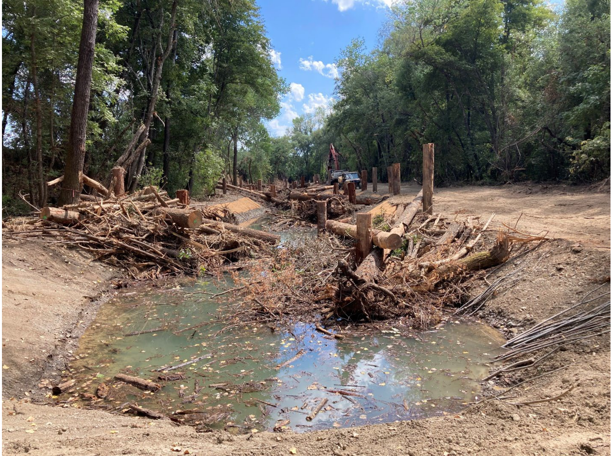
Photo 5.2. Dry Creek Ecosystem Restoration Project - Phase 1. Construction of habitat side-channel partially complete in Reach 13. August 29, 2022.
