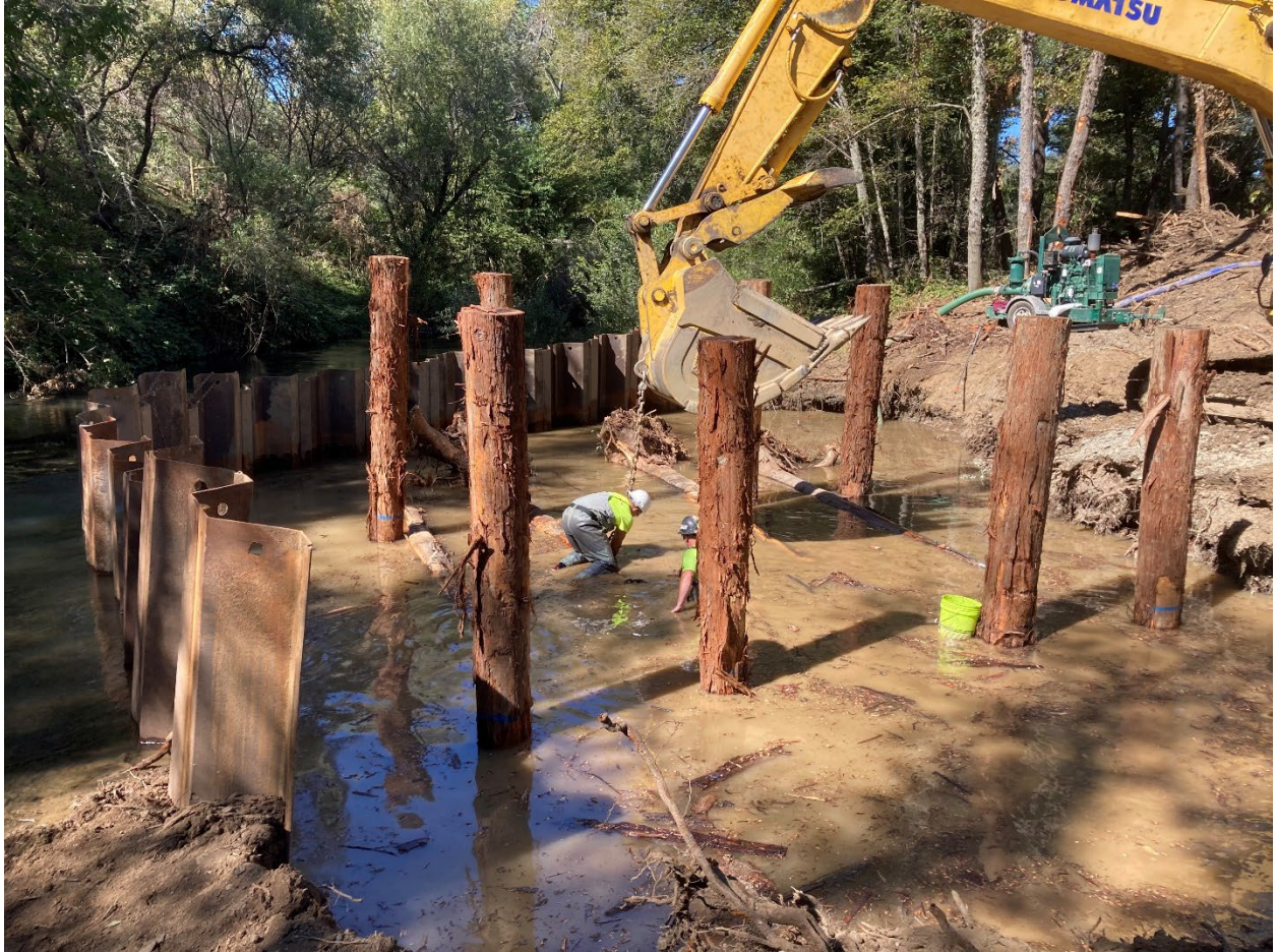
Photo 5.1. Dry Creek Ecosystem Restoration Project - Phase 1. Installation of an apex log feature at the inlet to a constructed side-channel in Reach 13. October 4, 2022.
