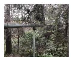
The influent carrier pipe at Sea Ranch Central Waste Water Treatment Plant is an 8 inch carrier pipe and 14 inch casing pipe that crosses the creek adjacent to the treatment plant. This pipe is nearing the end of its useful life and will be assessed for necessary rehabilitation, replacement, or other appropriate approach to mitigate the risk of pipeline failure.
