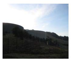
Sonoma Water's transmission system includes 18 steel water storage tanks at nine independent locations. Seismic assessment of the tanks indicate that some tanks may be vulnerable to tensile hoop overstress in the bottom course of the tank shell, resulting from the sloshing of water during a major earthquake. This project proposes to implement operational or design measures to mitigate those structural vulnerabilities.
