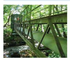
The 20-inch diameter Sonoma Aqueduct crosses Sonoma Creek at Lawndale Road off Sonoma Highway utilizing overhead spans (pedestrian bridge steel truss) with structural connections that make the pipeline susceptible to failure during a major seismic event. Liquefaction and lateral spread displacements will likely cause the pipeline to fail due to minor differential movement or settlement. The proposed project is a natural hazard reliability project that
