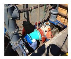
Mainline valve replacement at Jennings Avenue. Abandon existing location and acquire new location. The 36 inch mainline valve at Jennings Avenue is within SMART easement and thus Sonoma Water is unable to maintain the valve. The proposed new location will be downstream away from SMART easement and will include a mainline isolation butterfly valve of 36 inch diameter, and associated appurtenances.
