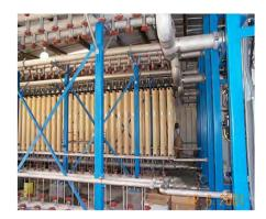
The Airport Larkfield-Wikiup Sanitation Zone Waste Water Treatment Plant treats waste water to tertiary standards meeting Title 22 requirements for disinfected recycled water. A critical element of the treatment plant is the microfiltration filters. These filters require periodic replacement of the filter media. This project will replace microfiltration filter modules at end of useful life.
