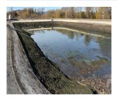
The Airport Treatment Facility does not currently have high flow or upset storage. In order to meet the winter inflow and possible bypass or upset without contaminating the tertiary storage ponds the facility must consider constructing an equalization basin. This may include additional features as the facility goes through a long term analysis.
