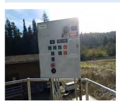
The Automation Project will remotely monitor and control wastewater storage between the Occidental lift station and equalization facility. Replace existing pump control panels and instruments at Lift station; install a slide gate and actuator, lighting and disconnect switches and PLC and communication at the Lift Station. Provide two valve actuators, flow meter, PLC and communication at the EQ Facility.
