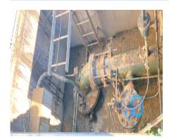
Electrical rehabilitation and pump install for Well #7 of the Russian River Wellfield located at the Mirabel production facility. Electrical is out of code and parts are not available so a new electrical panel is needed. Well #7 pumps water to infiltration ponds and Collector Well 1.
