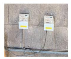
Chlorine gas (CL2) detectors inform staff, prior to entry, when gas is present within the tank rooms at Wohler and Mirabel. Current detector equipment is obsolete and the manufacturer does not support the product any longer. This project is to replace the existing antiquated CL2 detectors with up-to-date equipment.
