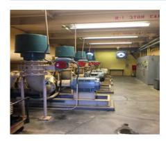
Wastewater treatment is a biological process which requires oxygen. Oxygen is supplied to the aeration basin by large high volume blowers through fine bubble diffusers. The District is pursuing a project to complete a comprehensive technical evaluation and based on the results of the evaluation the District plans to rehabilitate or replace the five existing 150 horsepower centrifugal blowers that are 40 years old and at the end of their useful life.
