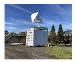
This project entails designing the installation of two radar units as part of the larger AQPI project. The radar units will be installed at a reclaimed pond located at the Airport treatment plant, and at a water storage reservoir located in Sea Ranch.
