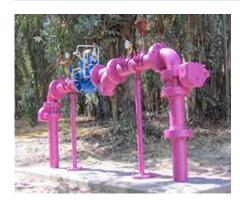
The Airport Larkfield Wikiup Sanitation Zone's recycle water system is the only mechanism to dispose of the highly treated wastewater that leaves the treatment plant. The Zone's current roster of recycle water users only use about one-third of the available water and additional users could improve the beneficial use. This project would construct two additional recycle water turnouts to supply high volume users.
