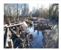
To address fish habitat issues associated with high flows in Dry Creek, as indicated in the Biological Opinion, this project will construct modifications designed to enhance fish habitat in Dry Creek Mile 6 while accommodating stream flows necessary to support water supply.
