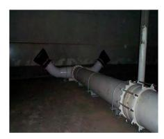
The Ralphine water storage tanks are located at Spring Lake Regional County Park, and are part of the Water Agency's Santa Rosa Aqueduct water transmission system. The project proposes to reconfigure piping at the four above ground steel water reservoirs at the Ralphine Tank farm to improve water circulation/turnover for enhanced water quality and address over constrained structural conditions to reduce the risk of damage during a seismic event.
