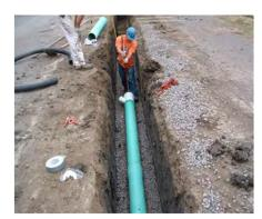
Construction of improvements to repair, rehabilitate, or replace portions of the collection and/or treatment systems that are deteriorated or have insufficient capacity for existing flows.
