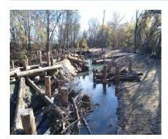
To address fish habitat issues associated with high flows in Dry Creek, as indicated in the Biological Opinion, this project will construct modifications designed to enhance fish habitat in Dry Creek Mile 5 while accommodating stream flows necessary to support water supply.
