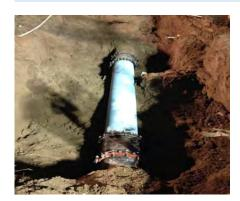
The Sonoma Valley County Sanitation District phase 5 project involves the replacement of approximately 8,245 linear feet of existing 21 inch and 18 inch reinforced concrete pipe trunk main in the SVCSD collection system with a larger sized trunk main to accommodate existing peak flows without overflows. This project is being built in response to a cease and desist order issued by the California Regional Water Quality Control Board to the SVCSD on June 10, 2015 (CDO No.R2-2015-0032).
