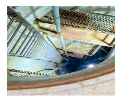
Reach Rods in Collector 5 are used to operate the lateral valves within the collector wells. This project will replace, in-kind, rusted, corroded, and worn out reach rods.
