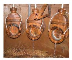
Underwater structures in the Mirabel collector wells are showing some evidence of corrosion and encrustation. In particular, some of the valve stem risers, brackets, and ladders show rust discoloration and, in some cases, scale and iron oxide nodules. Also, the ladders in Collectors 3 and 5 showed signs of more advanced stages of rusting near the bottom of the well. This project will replace the valves at Collectors 1 through 5.
