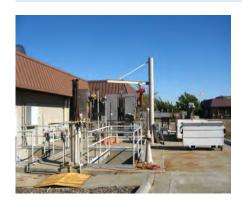
The headworks at Sonoma Valley treatment plant are reaching end of life. The mechanical screening and washing press equipment are requiring significant maintenance. The headworks are important as the first step in the process of treating wastewater and helps to remove large materials before continuing on to other processes. This project includes design, environmental review, and construction to replace the mechanical screening and washing press equipment.
