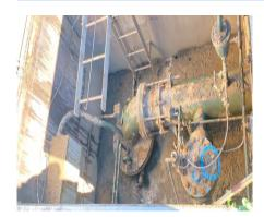
Project entails full rehabilitation of well, casing, pump, motor and electrical upgrade so that water can be pumped from the well to caisson 1 and/or infiltration ponds.
