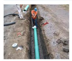
To prevent future Sanitary Sewer Overflows (SSO), like the one that occurred during the October 2021 rain event, where crews pumped approximately 200,000 gallons to minimize the SSO, this project proposes to replace the existing 6 inch force main (constructed in 1977) with a new 8 inch force main from the lift station through the Sonoma Marin Area Rail Transit's (SMART) right of way to Corona Road. Implementation is dependent on future grant funding.
