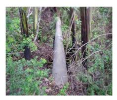
The 33 inch Petaluma aqueduct crosses the Petaluma River close to Highway 101. This crossing is vulnerable to liquefaction and lateral spread hazard with the potential to result in pipeline failure from a major earthquake. The project proposes to mitigate the seismic risk, which can be accomplished by relocating the pipeline such that it is below the lateral spread zone.
