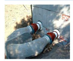
This project proposes to install a new vault around two existing shutoff valves located along the 20 inch and 24 inch discharge pipes at Collector 6. This new vault is required to facilitate needed repairs and maintenance on the valves.
