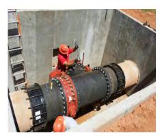
The existing 54 inch butterfly valve has failed and allows flow to the Cotati AQ when it should not be. This causes uncertainty with regulatory and operational functionality. The existing valve will be replaced with an improved valve that will allow flow control via automation and Supervisory Control and Data Acquisition (SCADA) control.
