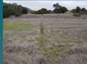
Looking across auxiliary spillway
