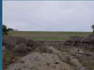
Looking at upstream face of dam
