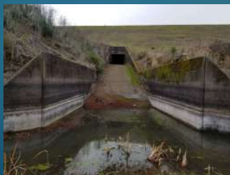
Looking at downstream face of dam
