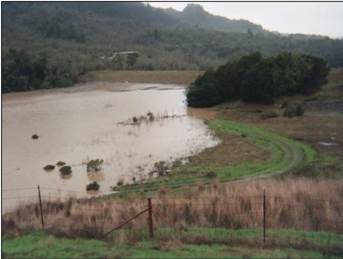
Dam crest for Matanzas Creek Dam is shown in the background. Auxiliary spillway crest is located several feet to the right of the shown access road. Photo courtesy of Sonoma Water.
