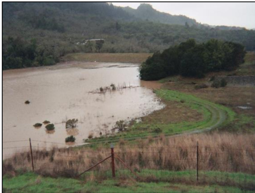
Figure 4-6. Matanzas Creek Dam reservoir water surface elevation after New Year's Eve 2005 rainfall event. Dam crest located in the background; auxiliary spillway crest located several feet to the right of the shown access road. Photo courtesy of Sonoma Water.
