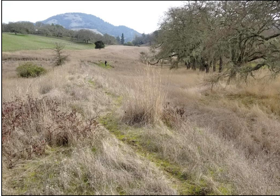
Figure 4-3. Lower section of auxiliary spillway (view is looking east towards upstream channel; photo is taken from top of constructed dike)
