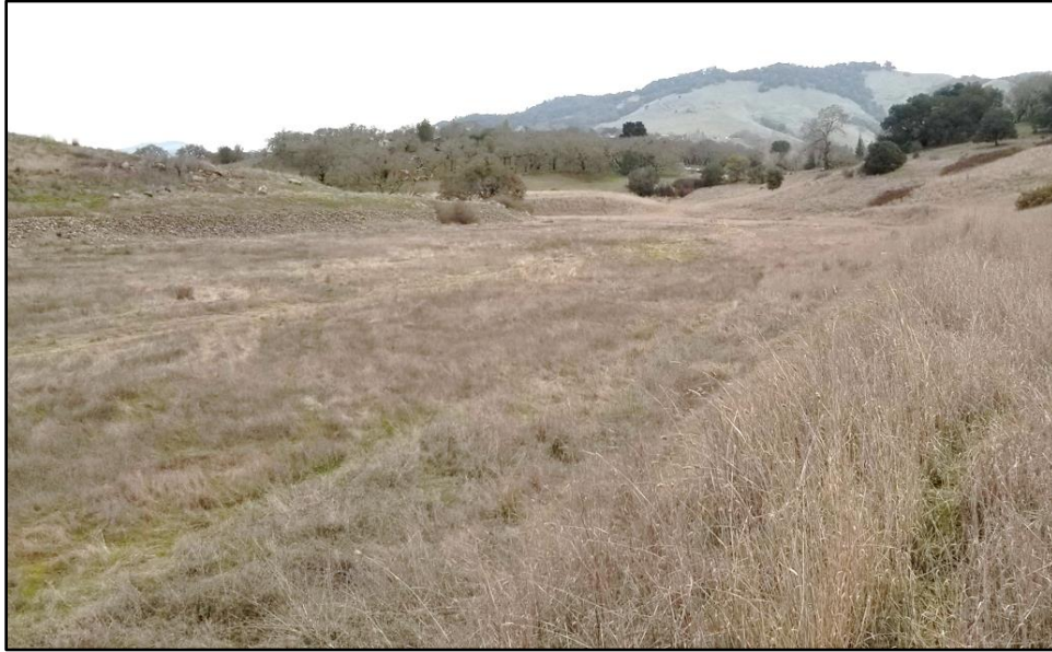
Figure 4-1. Upper section of auxiliary spillway (view is looking north towards downstream channel)
