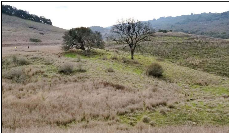
Figure 4-2. Middle section of auxiliary spillway (view is looking south towards upstream channel)
