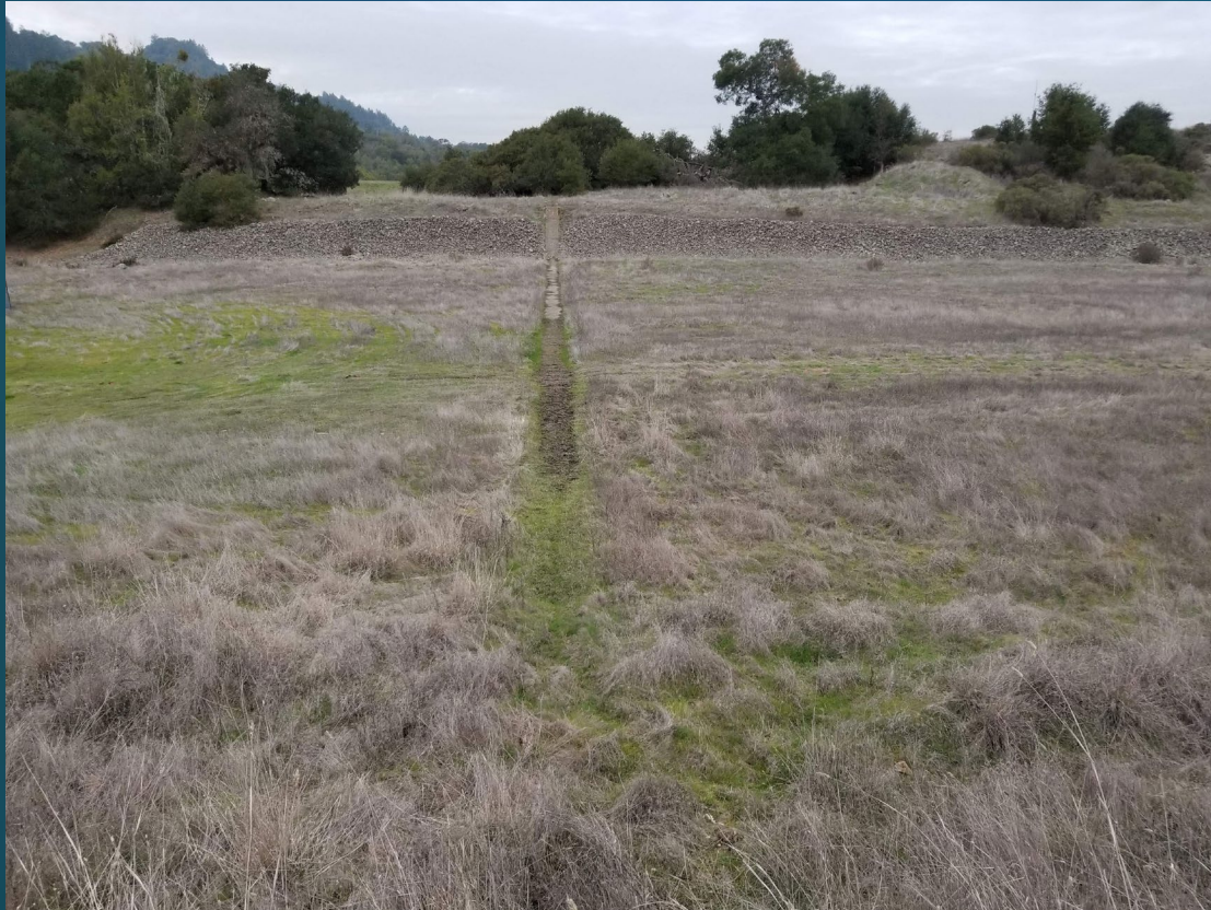
Auxiliary Spillway Crest (Weir)
