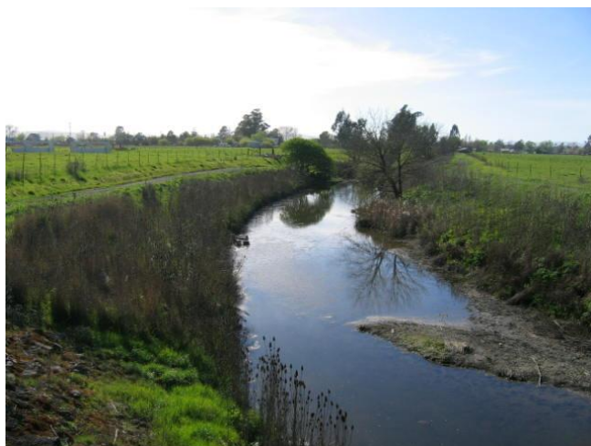
(b) Reach 4 looking downstream from first bend at railroad crossing; note wide channel, 10-12 ft below banks, with small point bar forming at inside of meander bend; riprap seen along outside bank (lower left); flow depth is 1-2 ft deep (March 14, 2007).
