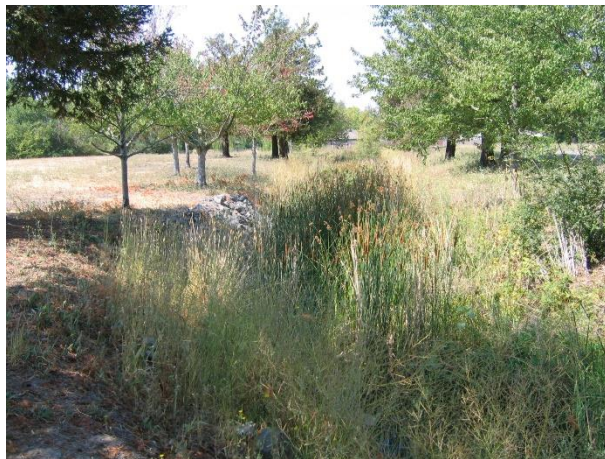
(b) Upper Reach 7 looking downstream: linear, trapezoidal channel is dry and choked with rushes and grasses. Several recent additions of rip-rap along banks (see left bank below the second tree) (August 2008).
