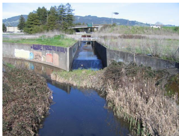
(a) Upper end of Reach 4, looking upstream to Todd Cr Reach 1 (left) and Wilfred Cr (at center); note drop structure at base of Wilfred Cr. and sediment wedge at confluence (March 14, 2007).
