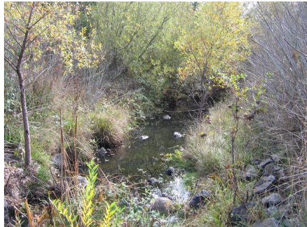
(d) Middle of Reach 3, looking downstream. Notice that the banks from the toe to the top are composed of large ungrouted rip-rap. This rip-rap is also found across the channel in many locations and appears to be functioning as grade control, and trapping and retaining sediments.
