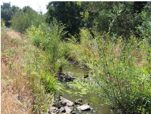
(c) Lower Reach 7 looking upstream. Eroded rip-rap extends into channel; several rip-rap banks appear unstable in many locations; water quality appears poor with brown stagnant water and extensive algal growth (August 2008).
