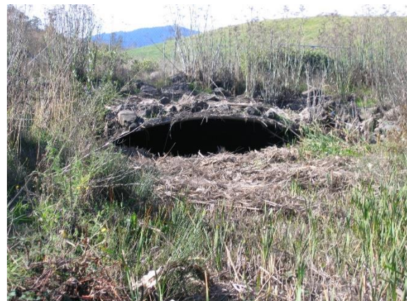
(d) Looking downstream at the culvert under Skylane Blvd. This aluminum arch is heavily impacted (as of 11/07) by sediment and cattail growth. It looks as though the culvert has lost at least ¾ of its capacity and the road bed is within a few feet of the top of the culvert. There is also a large sediment wedge on the downstream side of the culvert (May 13, 2008).
