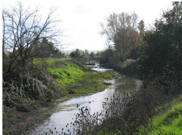
(d) Lower Reach 4 looking downstream to Millbrae Avenue; note large "D-shaped" bar along base of left bank where sediments collect on inner bend of channel (March 14, 2007).
