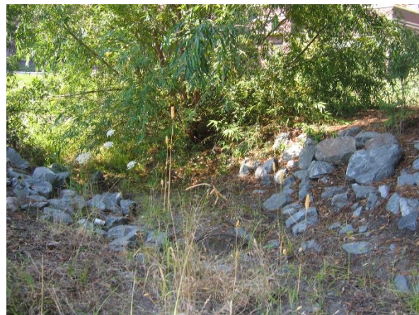
(a) Piner Cr. Reach 8 looks more like a seasonal swale than a typical flood control channel. Reach 8 was mostly dry in Aug 2008 with stands of cattails where the channel was still wet. The narrow channel includes rip-rap on the bed and banks (August 2008).
