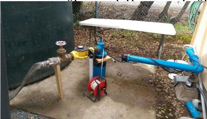
**Recovery (extraction meter between TW-6A and temporary storage tanks)**
