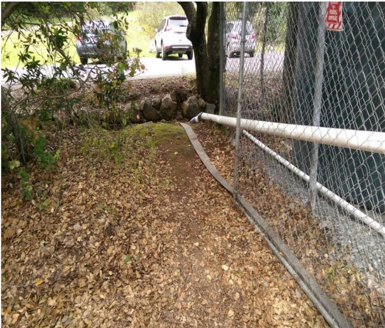
**Figure 4. Discharge Piping from Settling Tanks**
