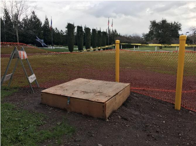
**Sonoma Water pipeline, connection valve box, vault for flow, sampling port, valves, and**
