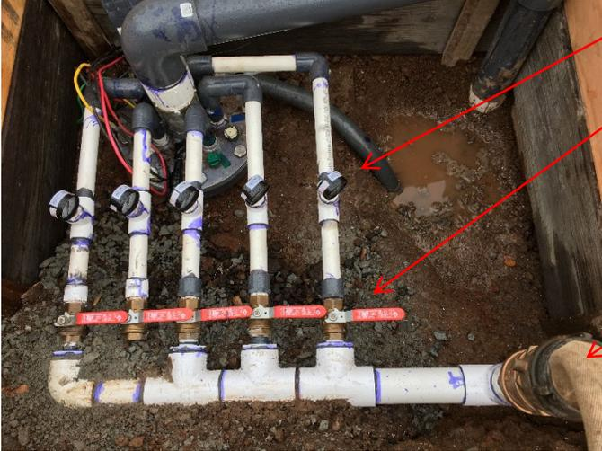
**Recharge (injection) tube with 3/4-inch orifice**
