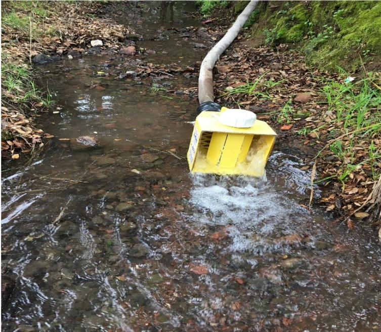
**Figure 5: Discharge of Water to Drainage Channel via Dechlorinating Diffuser**
