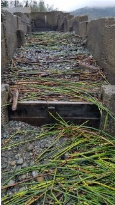
Figure 3-18. Cape Horn Dam Fish Ladder entrance showing accumulated sediment and debris.
