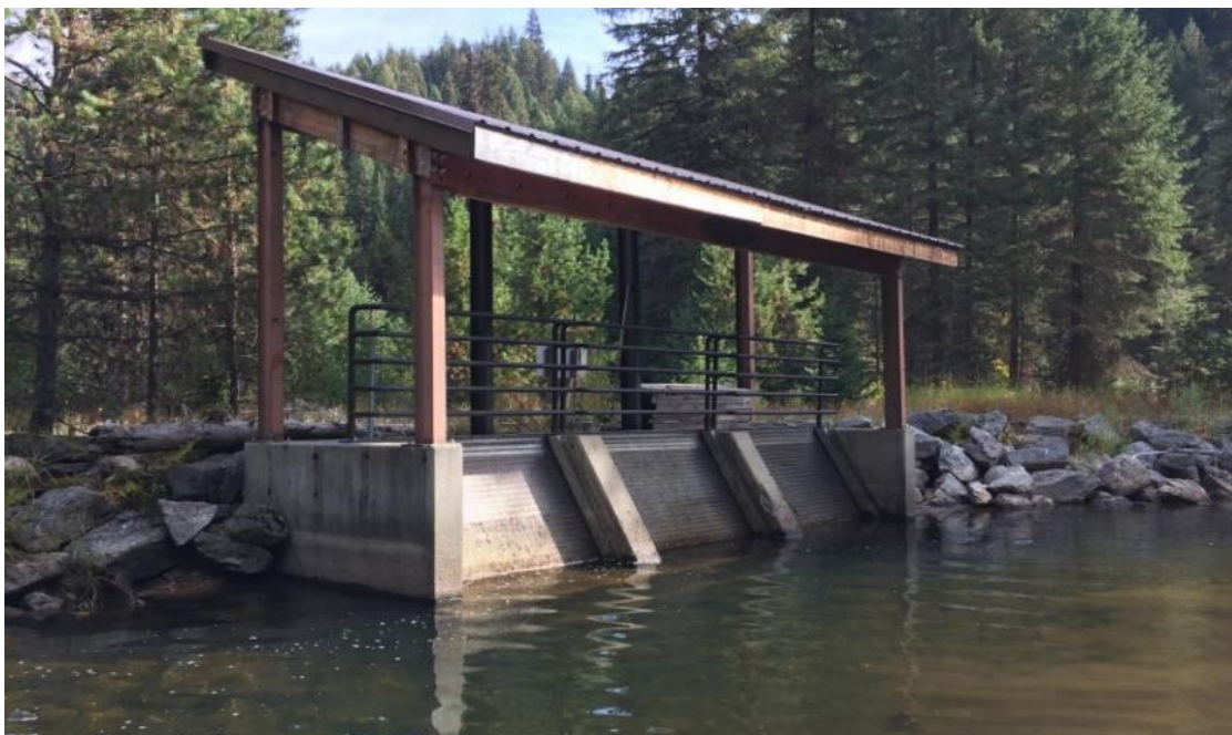
Figure 3-19. Inclined intake screen (passive cleaning).
