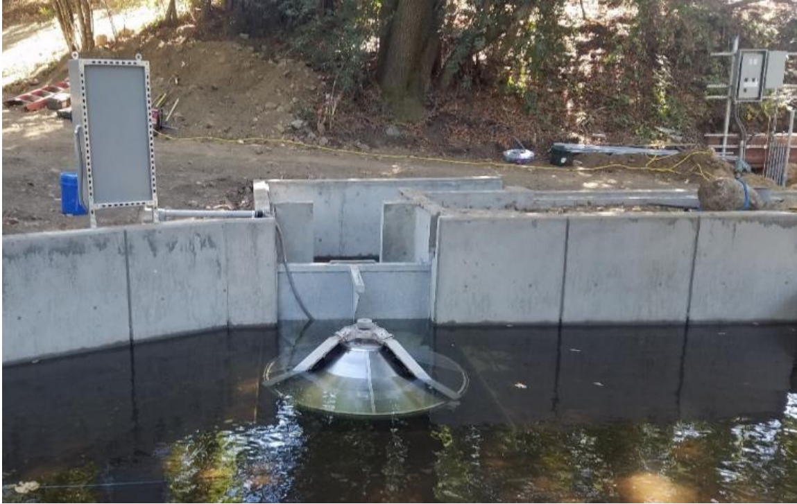
Figure 3-22. Cone screen on an adjustable bulkhead (photo courtesy of Intake Screens, Inc.).
