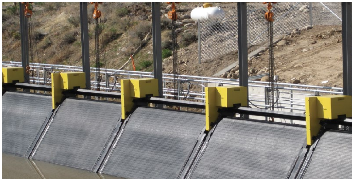
Figure 3-20. Inclined intake rotating screen (active cleaning).
