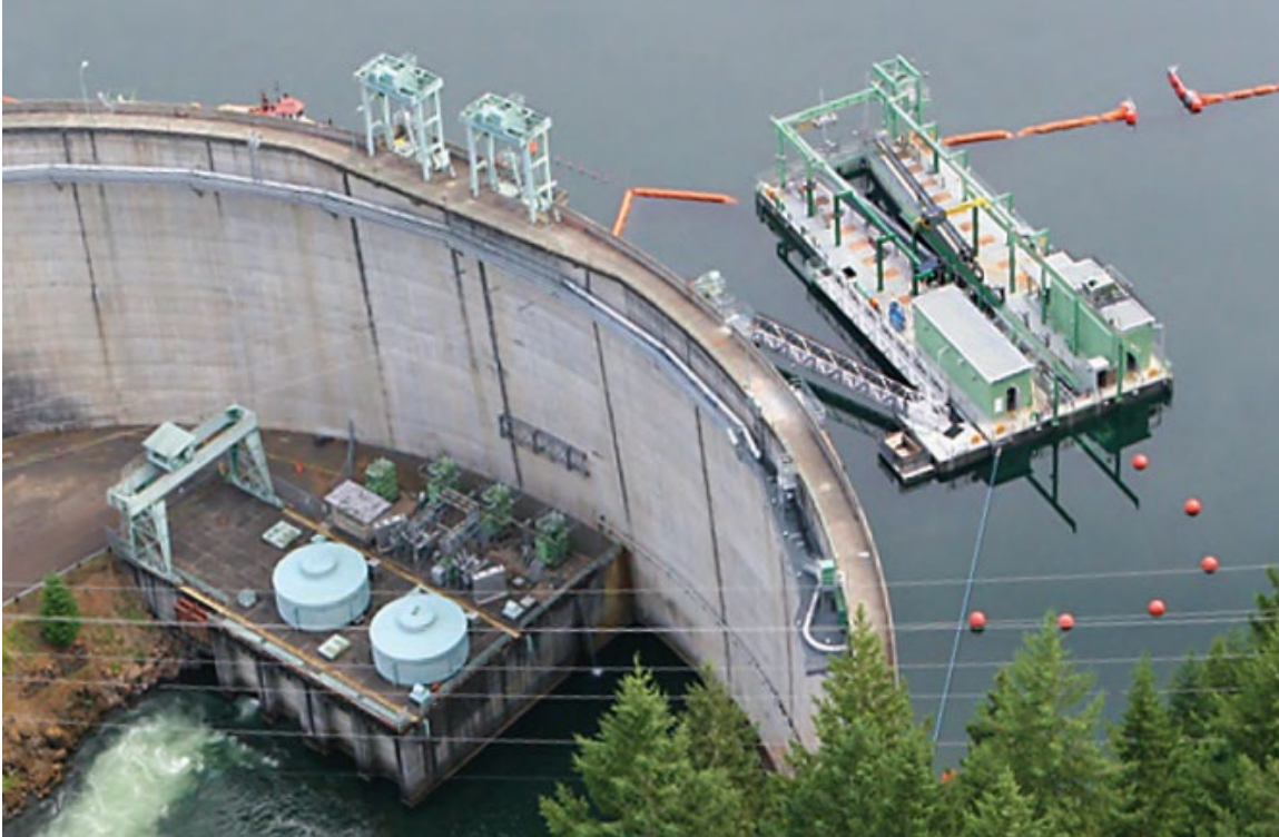
Figure 3-7. Floating Surface Collector at North Fork on the Clackamas River, Portland General Electric.
