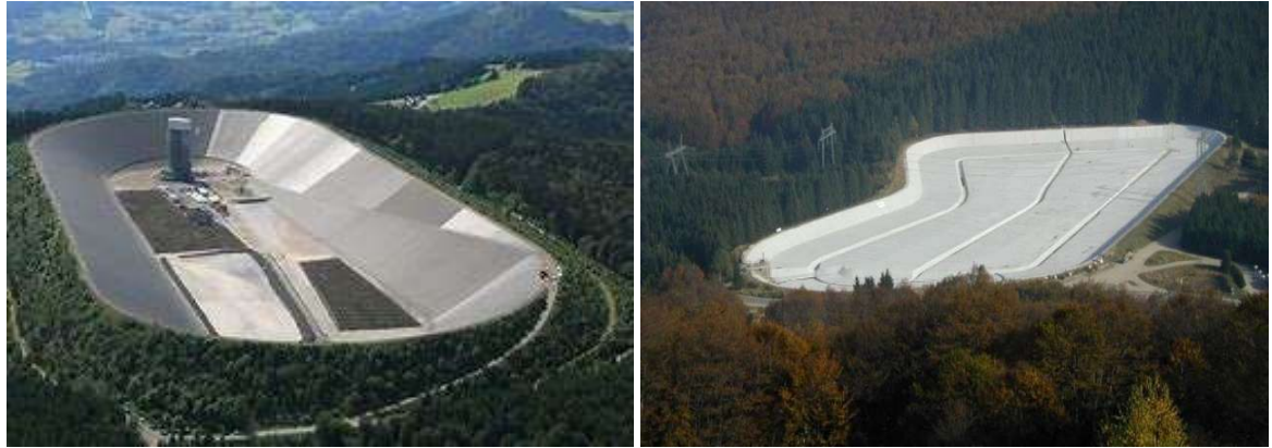
Figure 4-14. Example Liner Systems: WALO Asphalt (Left) and Carpi Geomembrane (Right)
