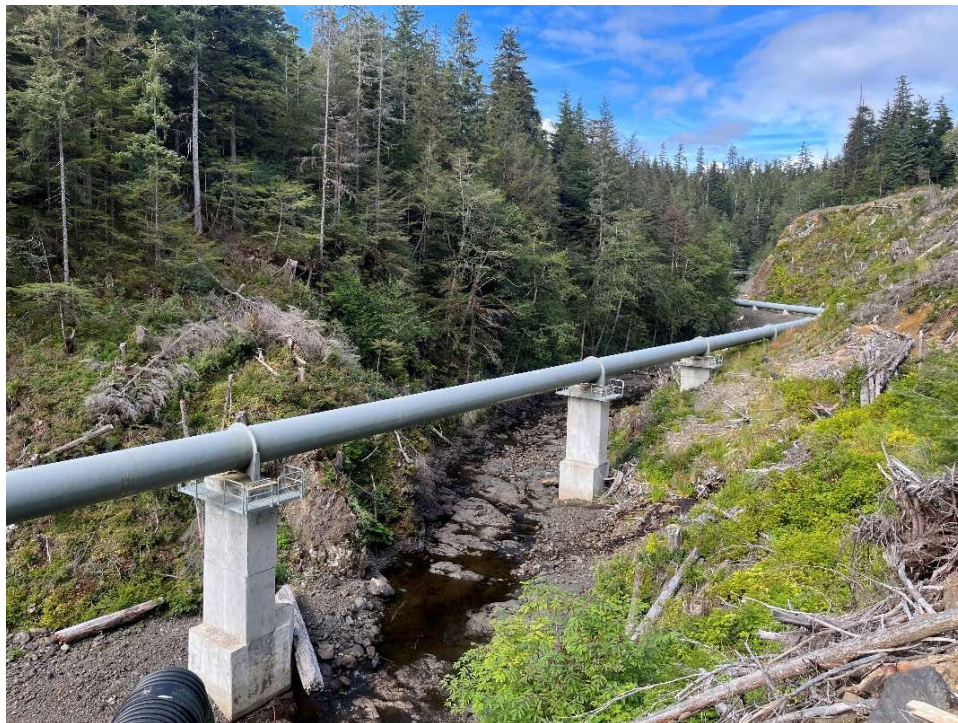
Figure 4-17. Example Surface Penstock Arrangement
